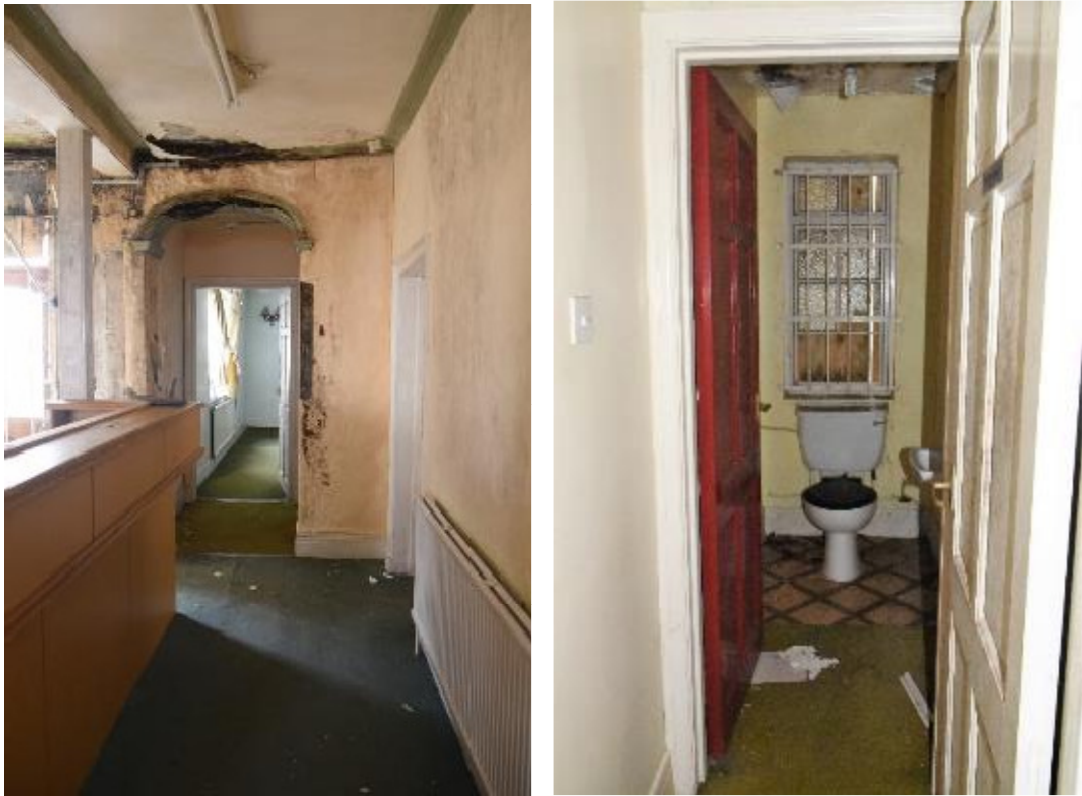
Figure 17 & 18 – image showing partial existing partitions to be removed.
