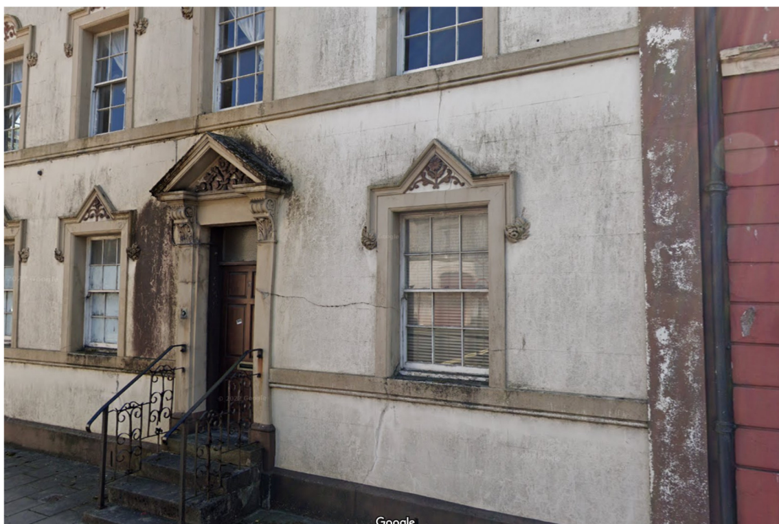
Figure 31 – Front elevation, showing crack between front door and window, and a crack from the window down to the ground, to be repaired.
