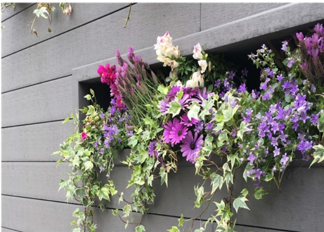
Cladding - Ecodec grey cladding
