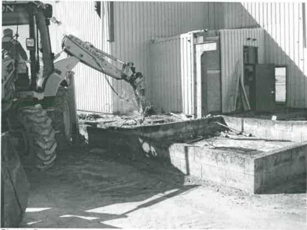
Plate 1: Breaking out concrete beneath location of former electrical transformer
