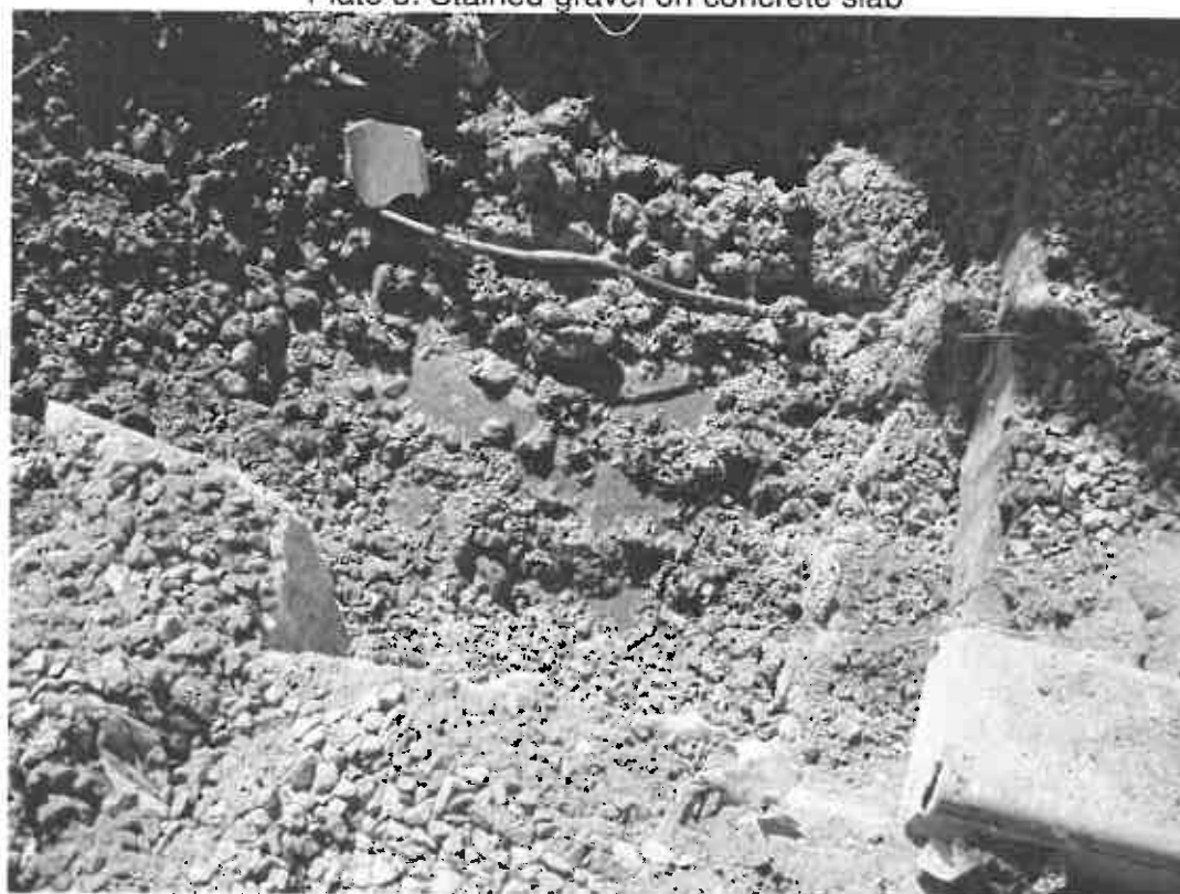
Plate 4: Evidence of oil contamination beneath transformer
