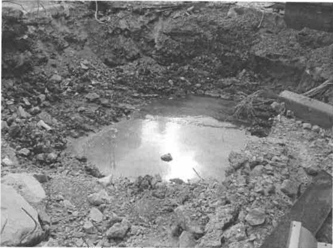
Plate 5: Excavation (water standing in base from existing drainage)
