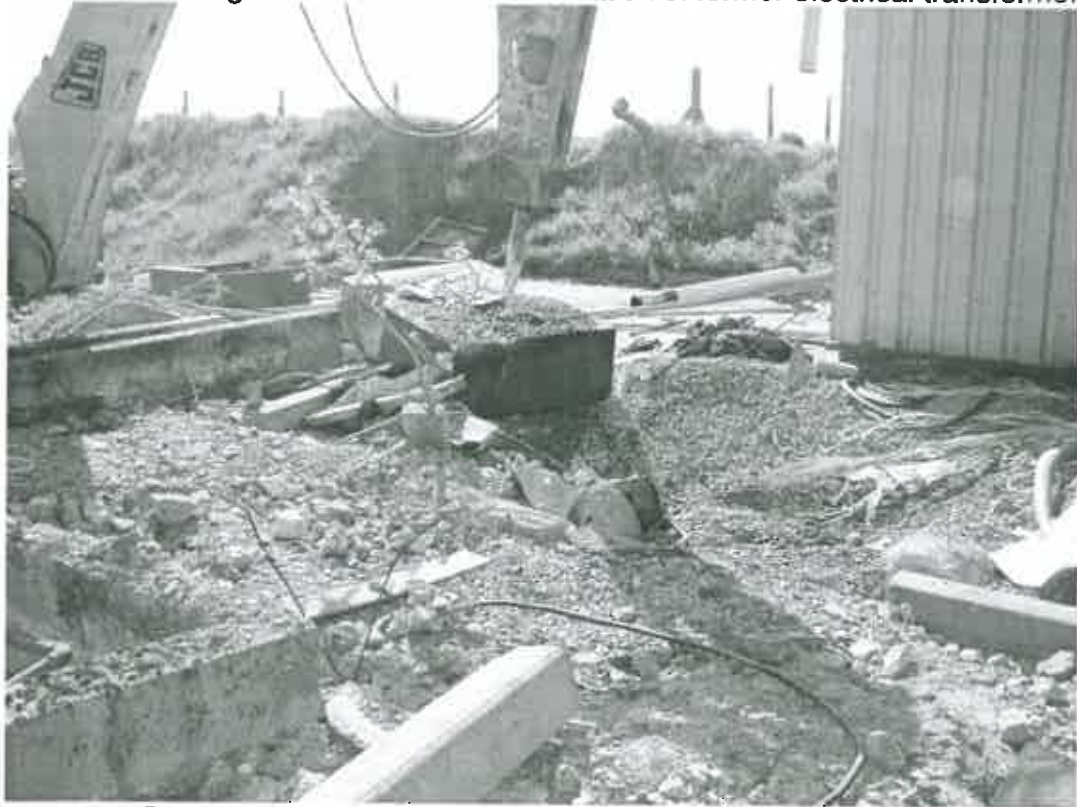
Plate 2: Removing concrete slab from beneath transformer
