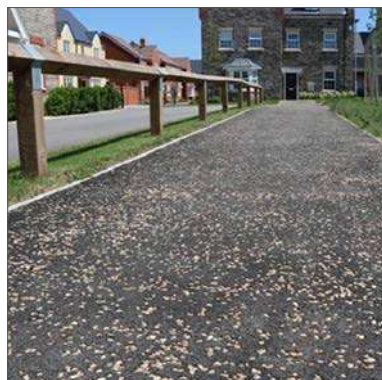
Aggregate blend incorporated within macadam surfacing - potential for contrasting streetscape to housing squares
