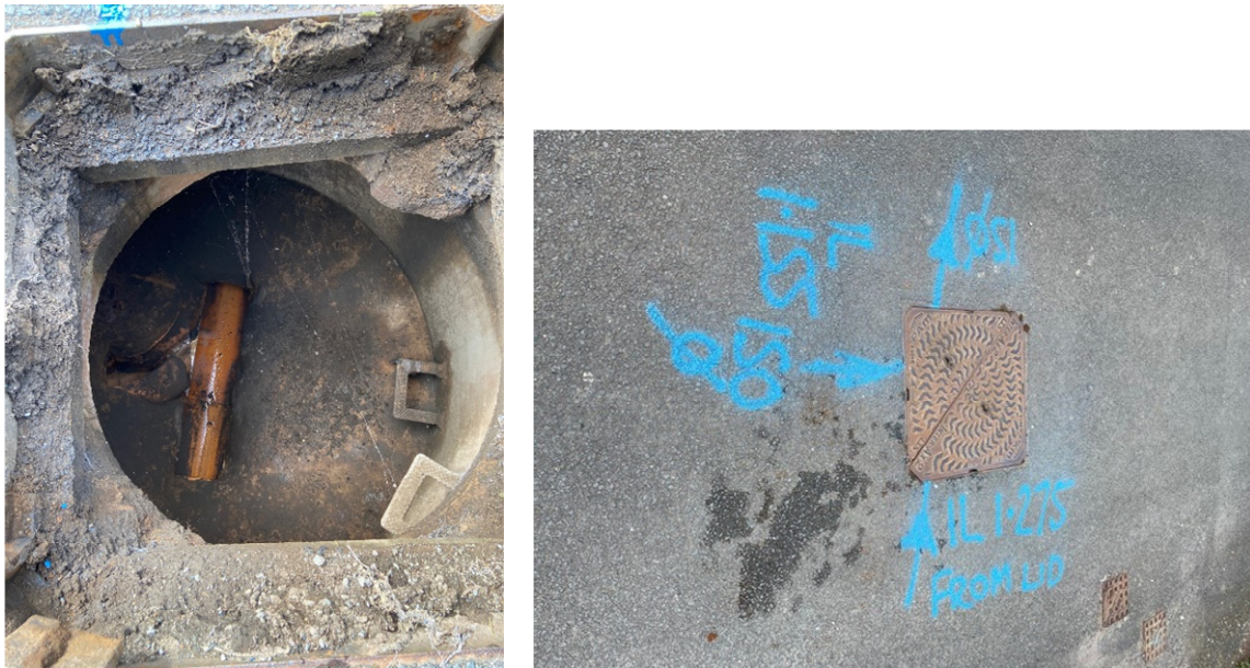
Figure 2 Ex. foul manhole in Nethertown Rd. Coords E:297168.299, N:511035.723
