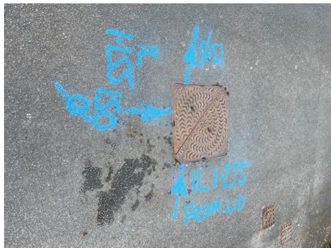
Figure 2 Ex. foul manhole in Nethertown Rd. Coords E:297168.299, N:511035.723
