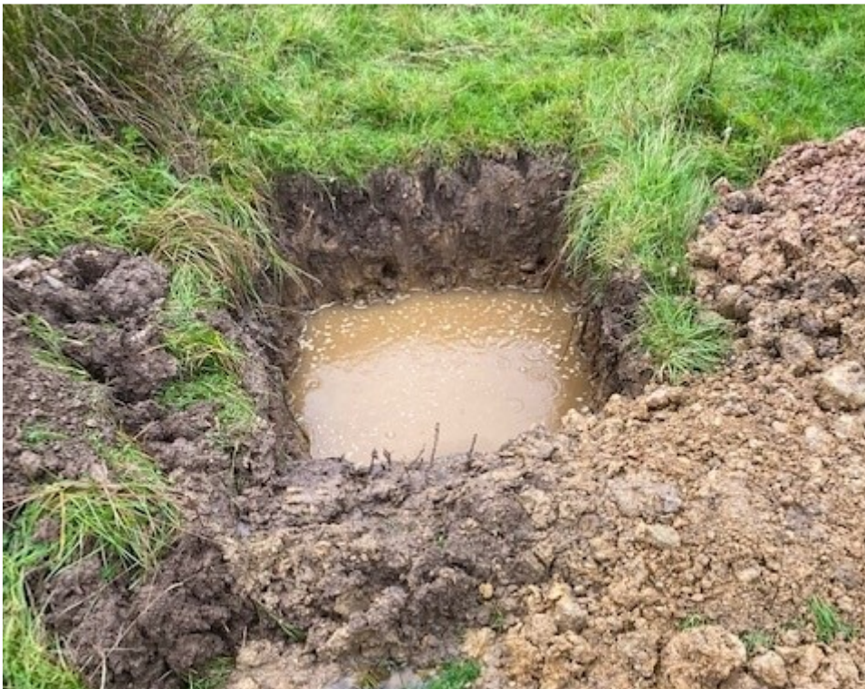
Figure A3: Photograph of a trial hole dug on site (Trial Hole 1)
