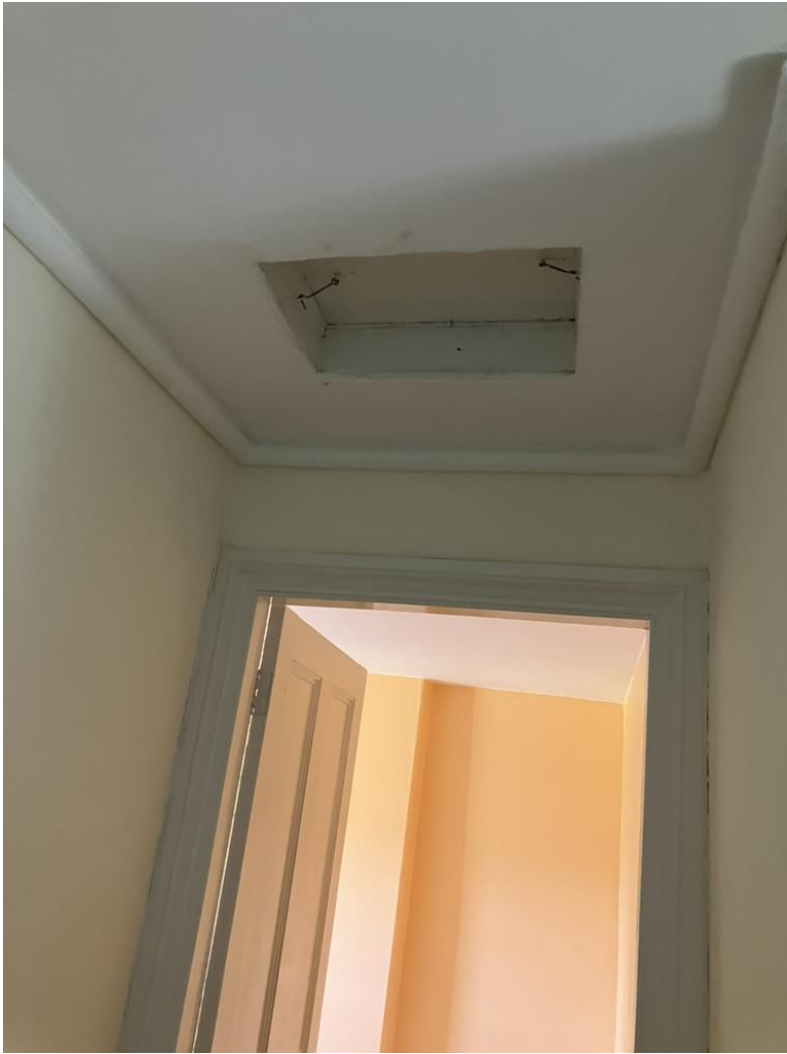
Ceiling hatch to Second floor to be removed and enlarged in same location
