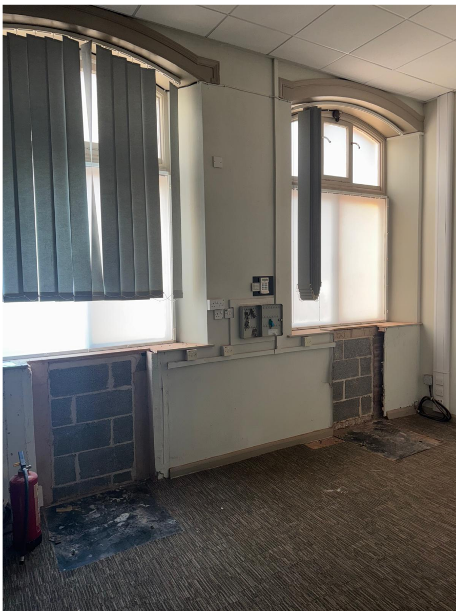
Internal view of original building frontage – blockwork wall infills show location of cash machines now removed and sandstone repairs completed to outside. Suspended ceilings to be removed.
