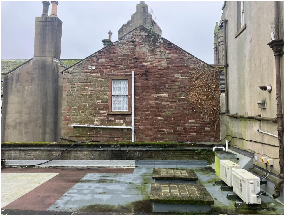
External views looking across the single storey flat roof element of the building below the old offices. Concrete / glass rooflights provide daylight into the depth of the ground floor plan.
