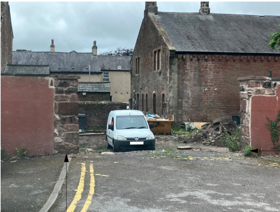
existing sandstone wall made good and returned
