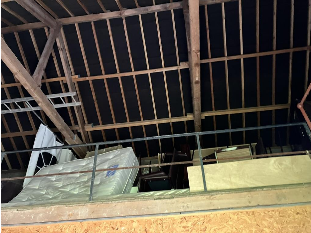
New roof in barn with roofing felt
