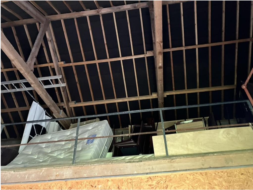
New roof in barn with roofing felt
