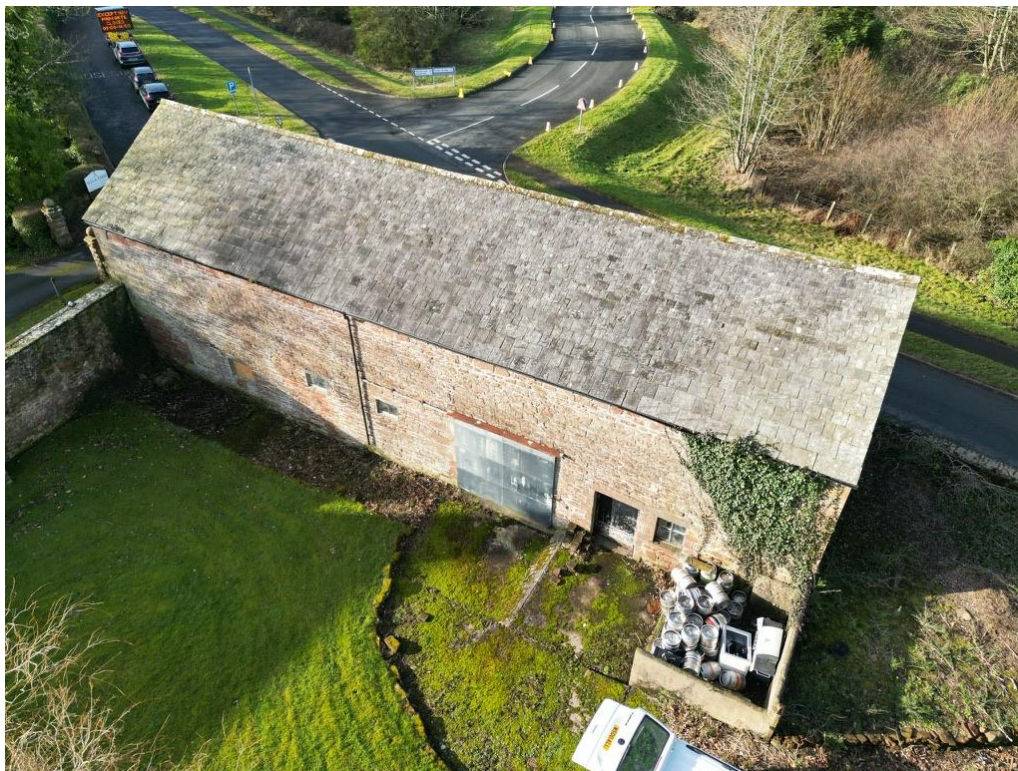
Aerial view of re-slatted roof
