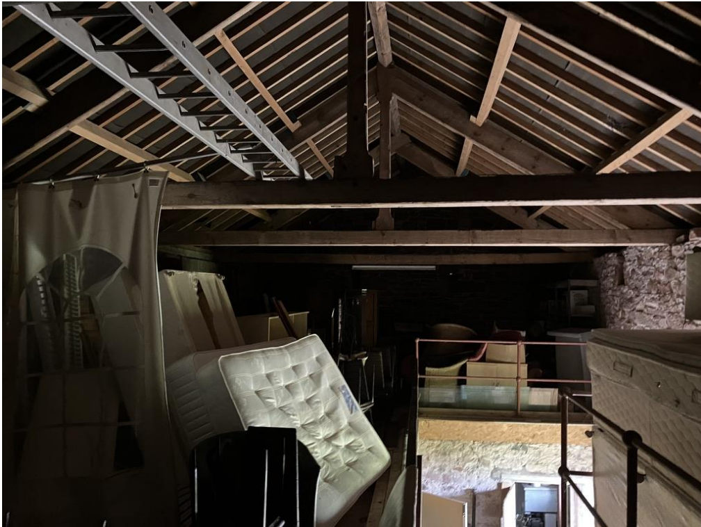
View through upper floor with trusses sat on re-built walls
