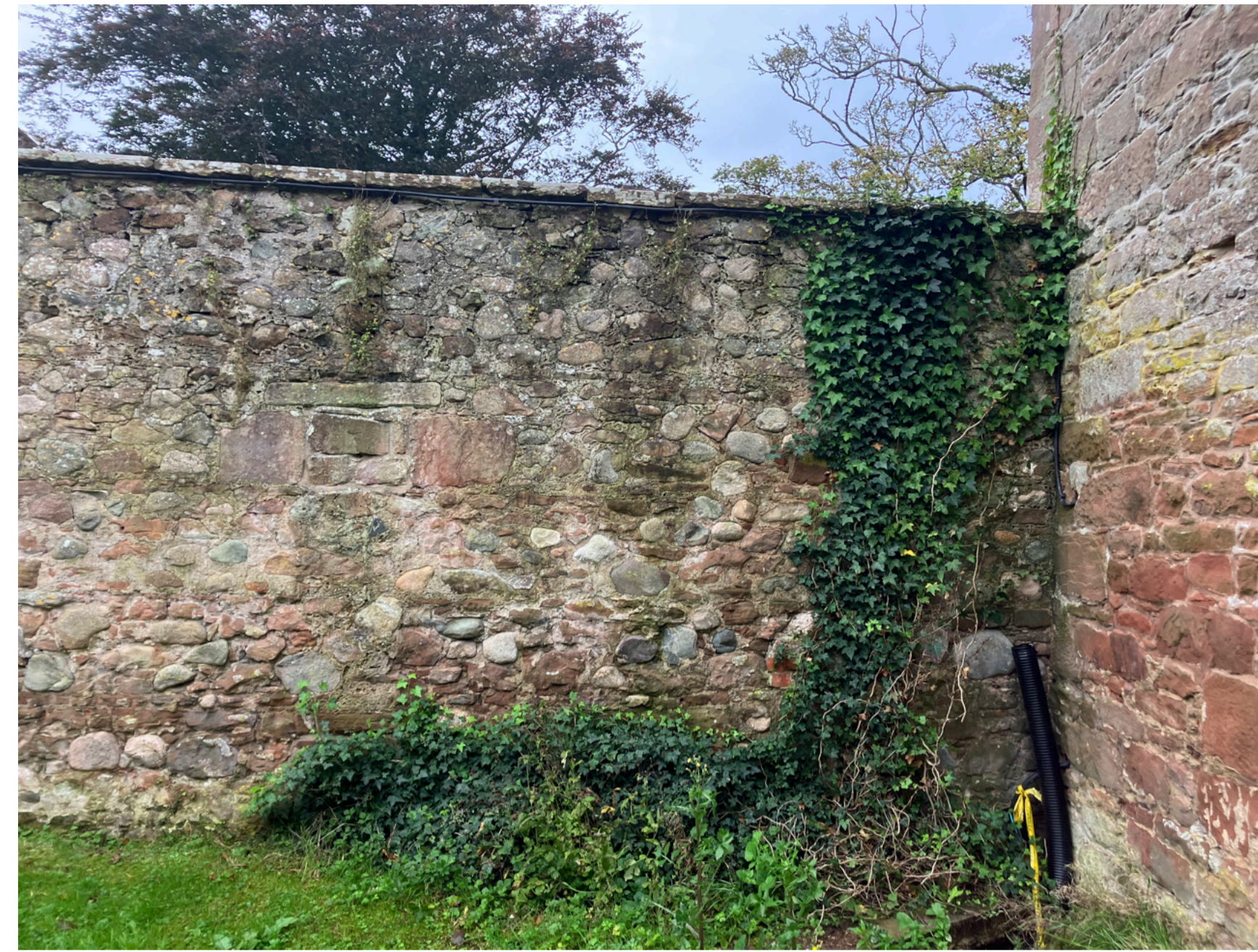
INTERNAL VIEW OF BOUNDARY WALL TO BARN ( NORTH )
