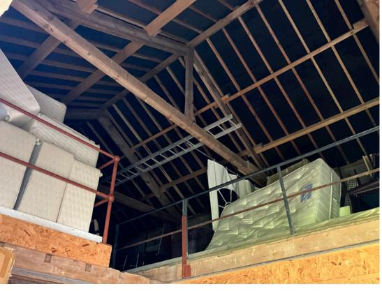
existing roof trusses retained - new timber purlins and roof timbers - roofing felt previously fitted by Sellafield
