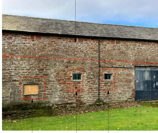
existing lintol - concrete lintol removed, propped and lifted in sandstone
