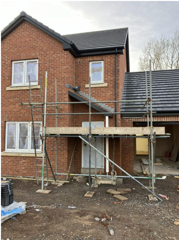
Pre-cast Cills to front and rear – uPVC fascias and soffits in black
