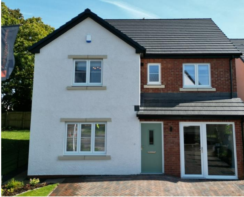
Pre-cast lintols to window heads
