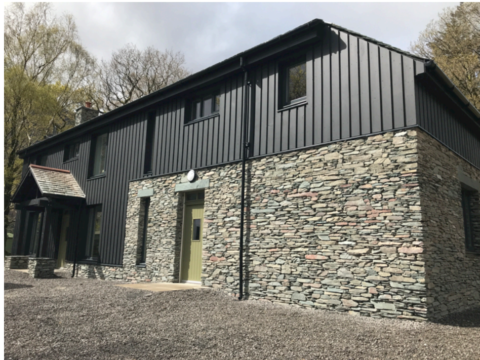
black stained larch installed in Buttermere
