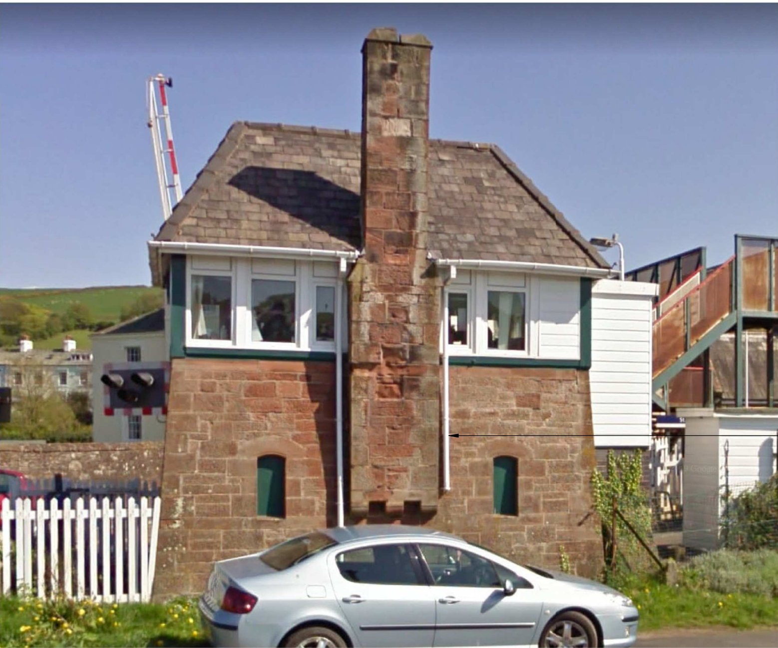
P1 - PHOTOGRAPH OF RWP TO BE REPAIRED
