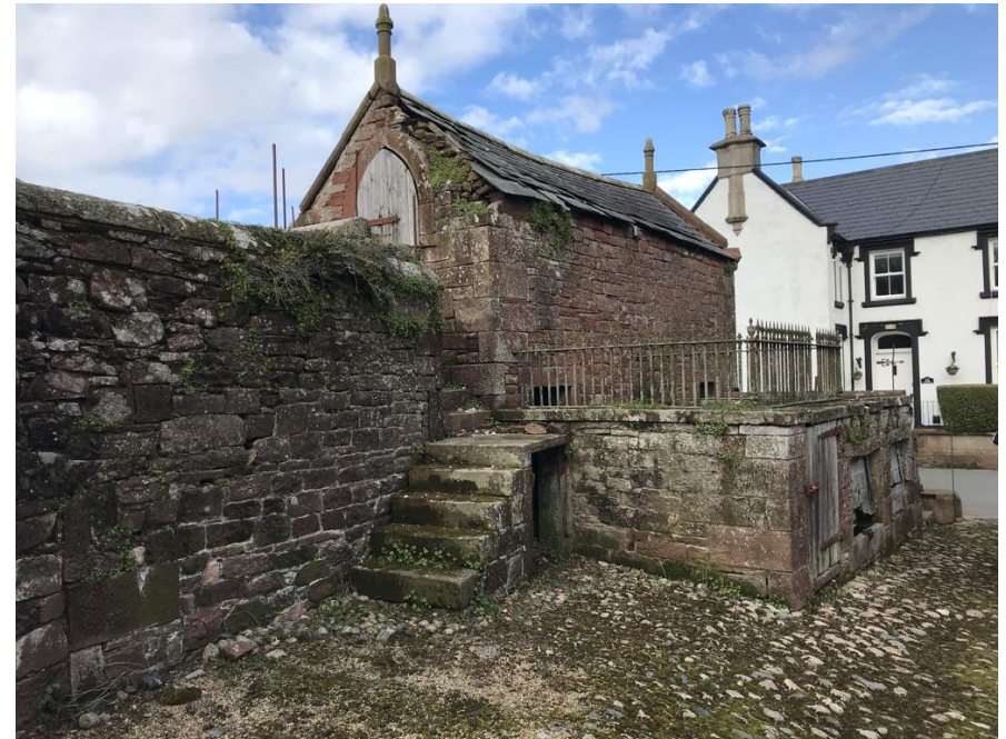
Rear view of Piggery showing decay in stonework ( retained on site ) and loose / slipped slates as a result of timber failure.
