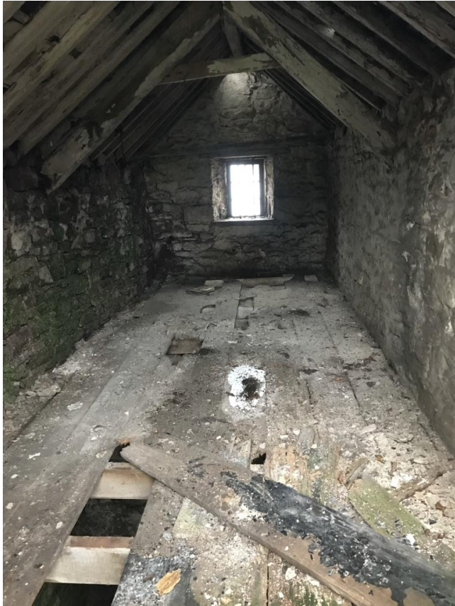
Internal view of upper floor level with decayed floor boards and joists
