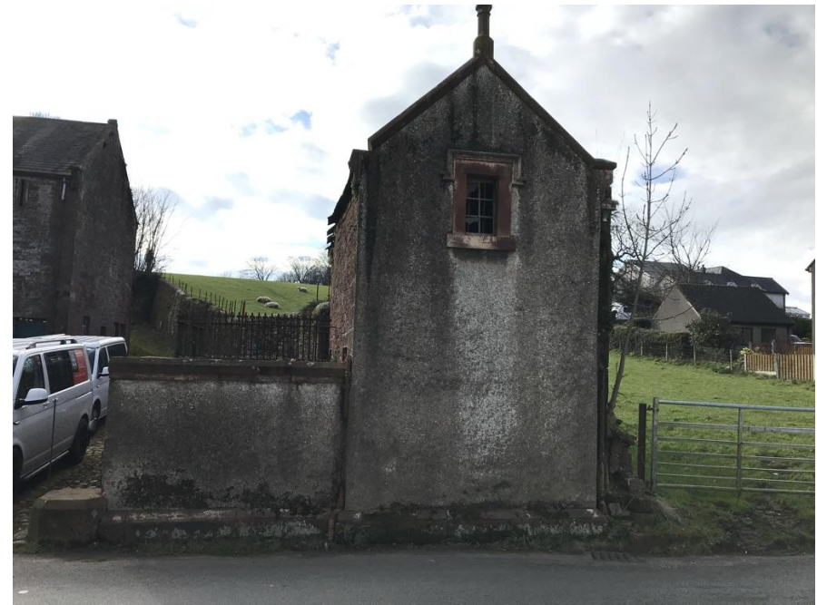
Front elevation with spar dash to roadside and hooded mouldings to gable window
