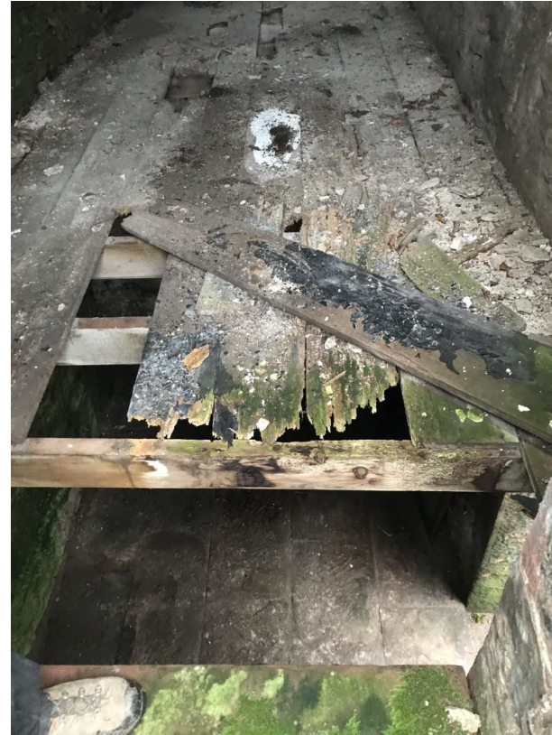
Joists and flooring missing at entrance due to water penetration below the original door
