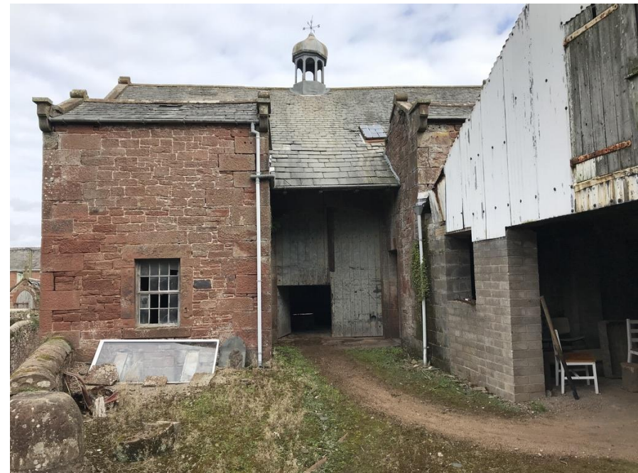
View looking East, modern gin house wall to be moved back to allow view of existing symmetrical turreted sandstone rear outriggers
