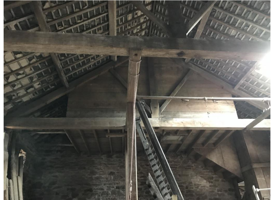
Double height barn with kingpost truss and pigeon loft bearing on truss chord
