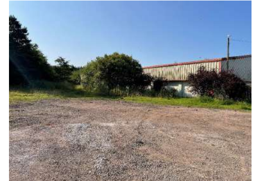
Rear of centre – space for expansion
