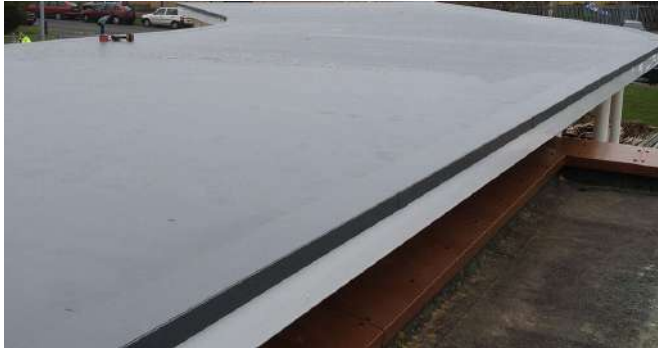
Single ply roofing
