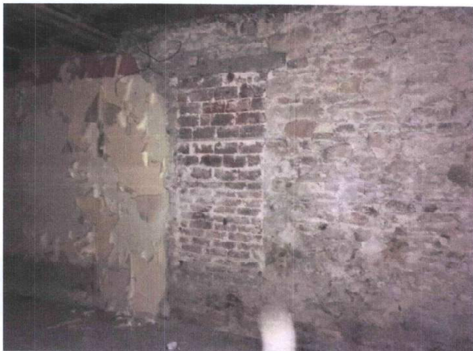
Plate 8. Evidence of an infilled window in the longitudinal internal dividing wall through the middle of the former Chinese restaurant
