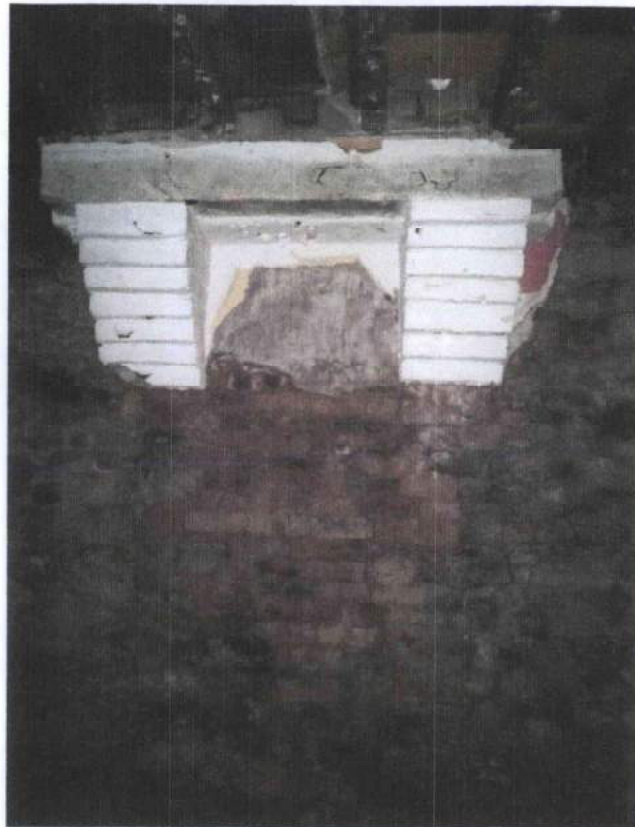
Plate 9: South interior wall of the ground floor of the former Chinese restaurant showing brick infill within a rubble wall and a hearth support for the first floor
