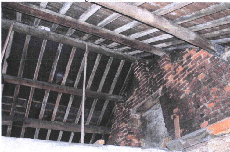
Interior view of roof looking south east.
