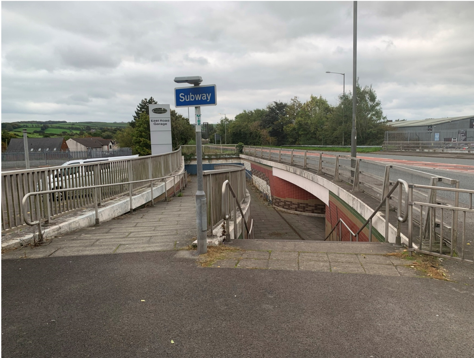
Picture 4 – looking south along the western boundary at the pedestrian subway.
