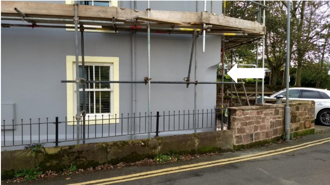
Figure 43 Stopped chamfer at the corner of Fleatham Farmhouse. This was probably either to allow space to pass behind the dwarf wall, or it predates the wall and was originally to protect the corner from passing carts etc.
