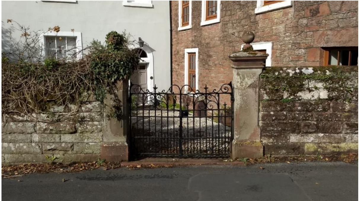
Figure 99 This property on High House Road features impressive squared rubble walling, with grand gate piers and a very attractive gate forming a feature.
