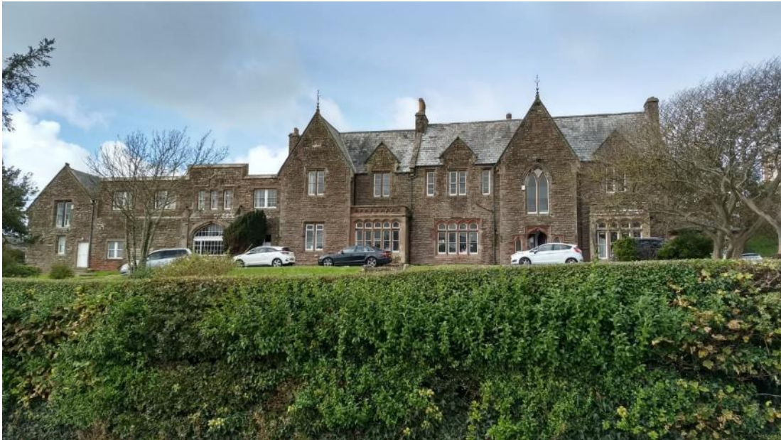
Figure 29 Abbots Court, outside the conservation area but within its setting
