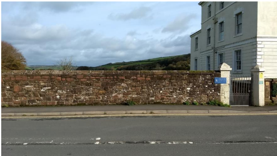
Figure 104 Characteristic red sandstone walling with triangular copings near the station and Grindal House
