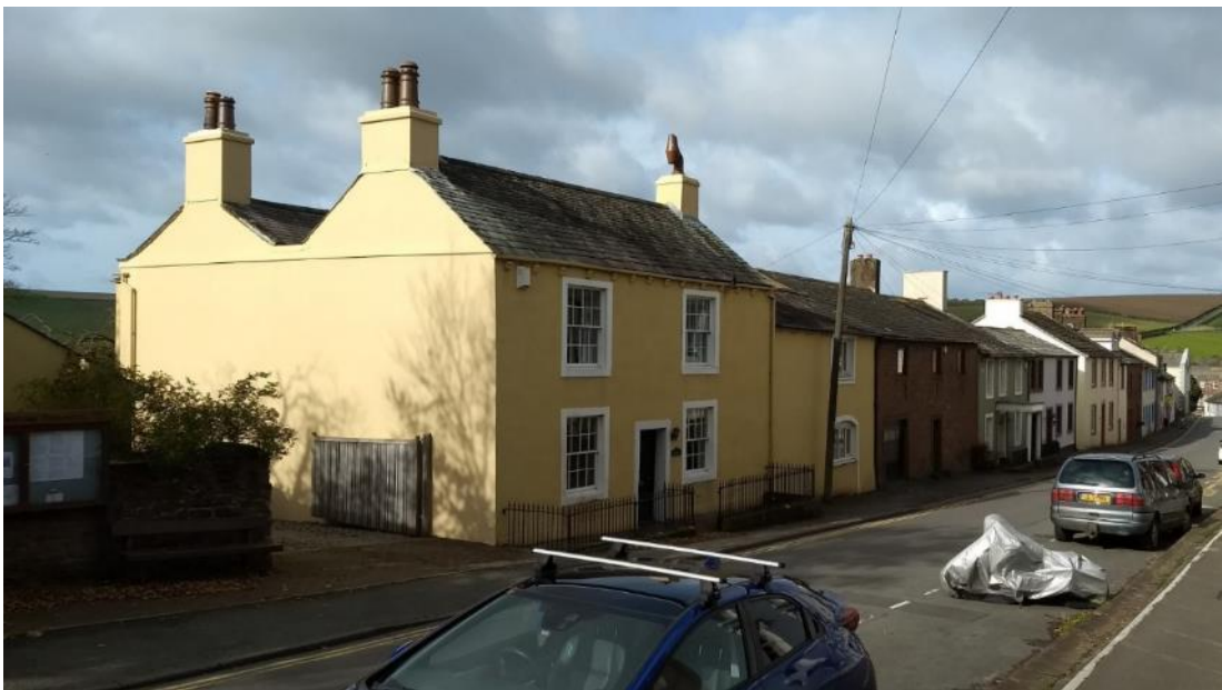
Figure 64 Orchard House (115 Main Street) is a grade II listed late 18 th or early 19 th century house with a distinctive late Georgian "double plan", consisting of two pitched volumes with a valley between them.
