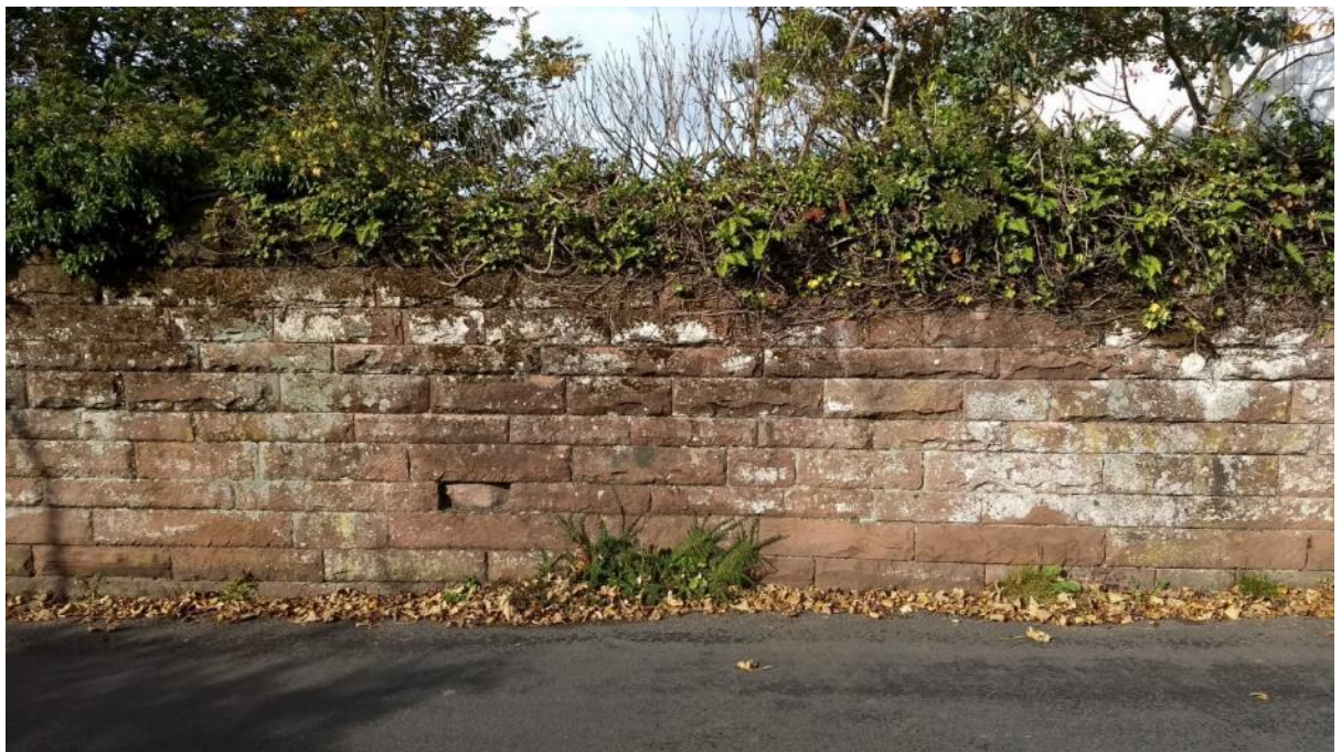
Figure 100 Squared red sandstone rubble wall with half-round copings and vegetation on High House Road. Though the vegetation is a key part of the sensory qualities of this area, it can also damage masonry if left unchecked.
