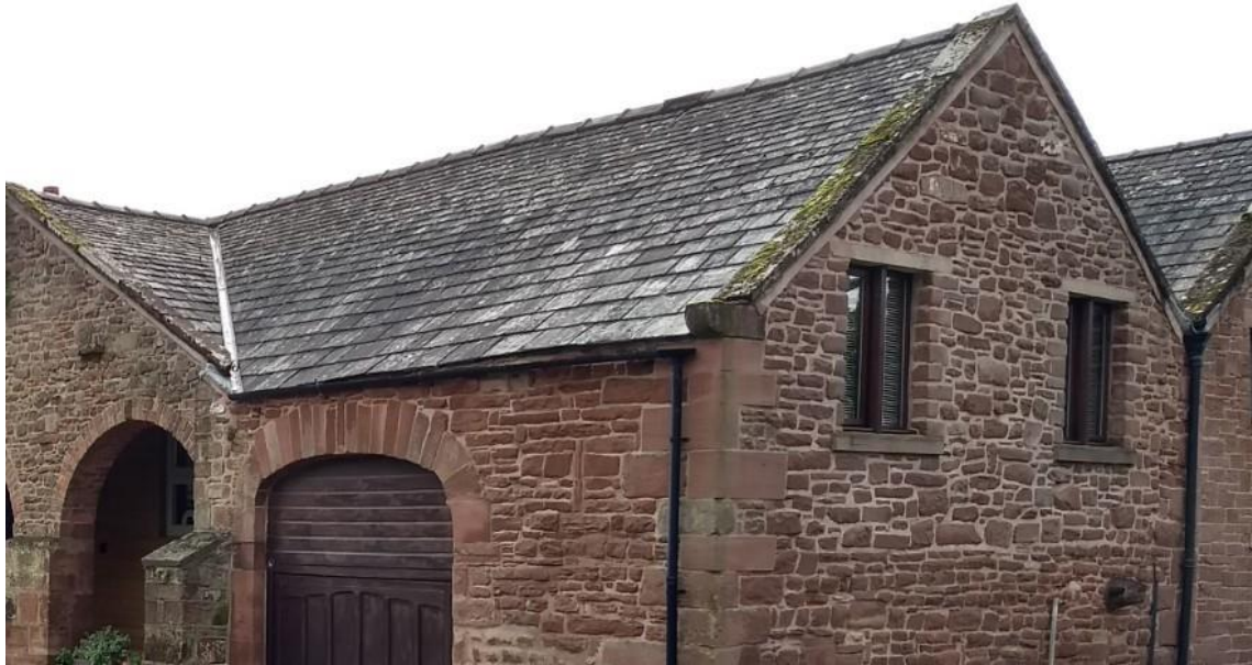
Figure 81 Lakeland slate roofs are characteristic of the conservation area, and sit well with red sandstone or coloured stucco. Their replacement with tiles is rarely beneficial to the area's appearance, and normally resisted.
