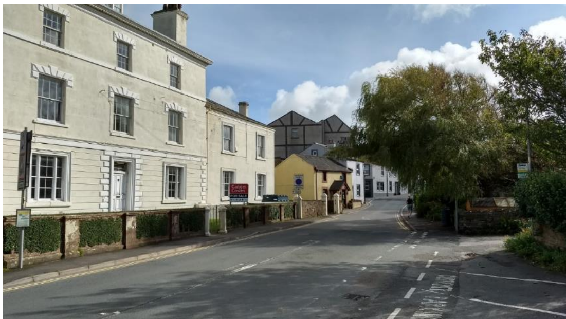
Figure 9 Grindal House, a grand and somewhat elaborate Victorian building that is listed grade II, as are the boundary walls in front of it. Together, these create a very positive impression. Though various poor quality extensions to the rear have had a detrimental effect, these are fortunately fairly hidden from Main Street.
