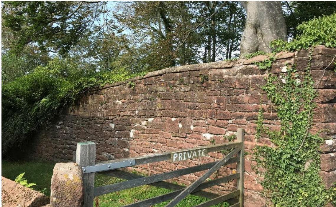
Figure 97 One of the many red sandstone walls that characterise St Bees' conservation area on High House Road. Dressed rubble with half-round copings. Many of these bound the gardens of large properties or define snickets, as here, leading up the side of Grindal Place.
