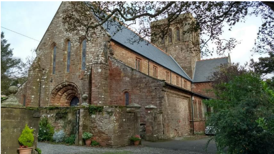
Figure 20 The priory viewed from the south-west, showing the Norman west doorway
