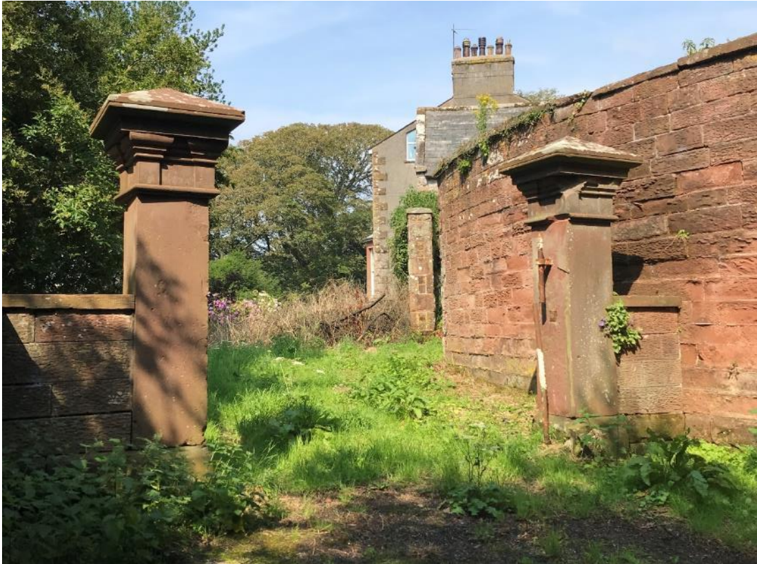
Figure 33 Grand red late 19 th century sandstone gate piers and walls at the entrance to High House. Parts of iron gate hinges remain, but the gates themselves are gone.
