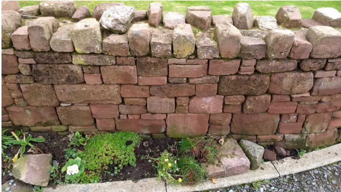
Figure 101 This "cock-and-hen" walling is only a few years old, but it is a well-executed example of a locally distinctive typology. Its use on Abbey Road successfully frames the street and entrance to a house.
