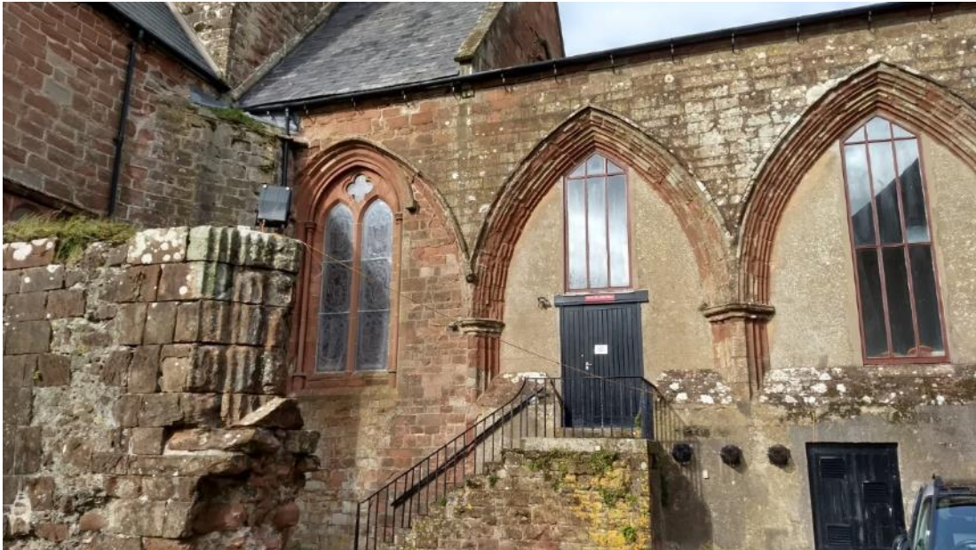
Figure 19 The Old College Hall, viewed from the south. The fluted masonry in the foreground is likely part of the current building's original 12 th century phase.
