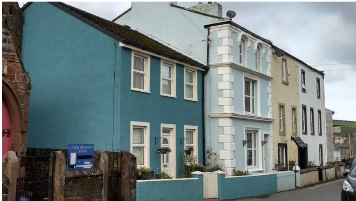
Figure 80 Coloured render also has a strong tradition in St Bees, with buildings providing uplifting splashes of pastel or earthy hues that contrast well with the deeper qualities of red sandstone. Painted render also has the ability to show off more ornate detailing, as is the case here with the paler blue house.
