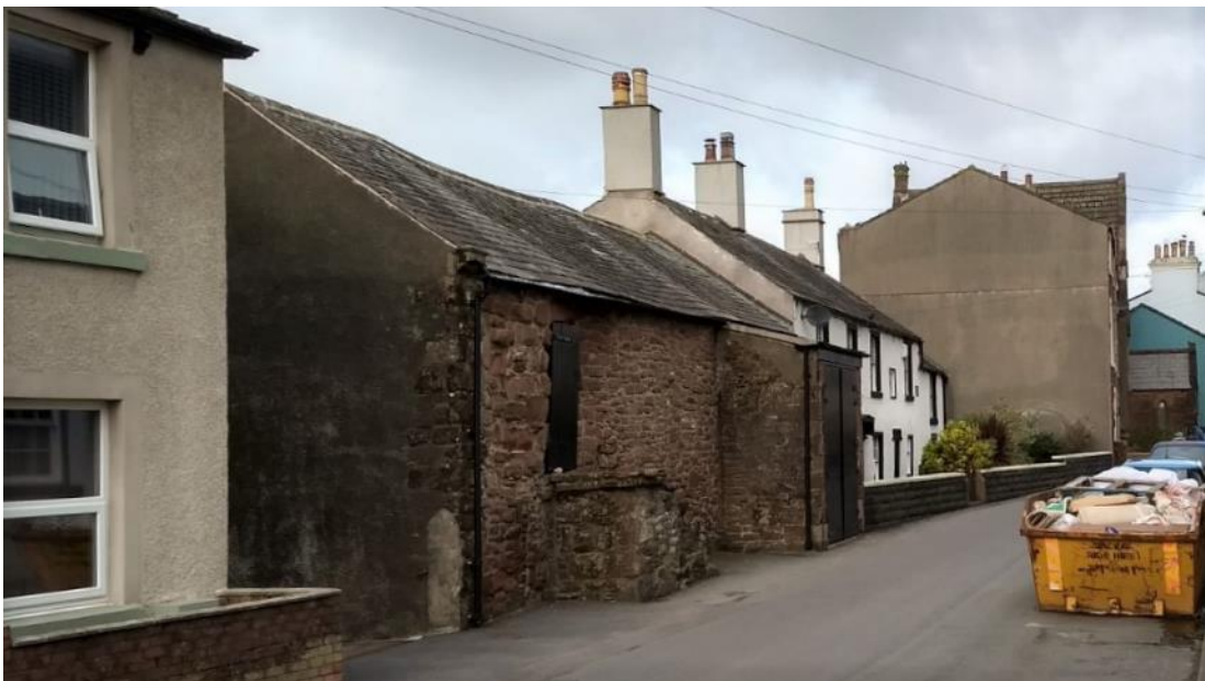
Figure 72 Fairladies Farmhouse and its attached barn, which is also grade II listed
