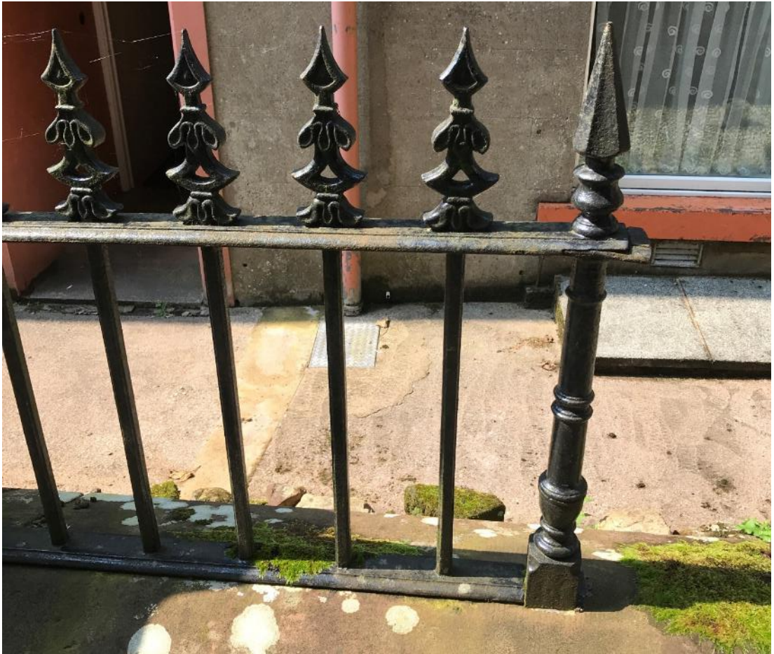
Figure 35 Historic iron railings and sandstone wall surviving outside Meadow House, in combination with unattractive concrete additions, either associated with the building's use as a school sanitorium or its later conversion into flats.
