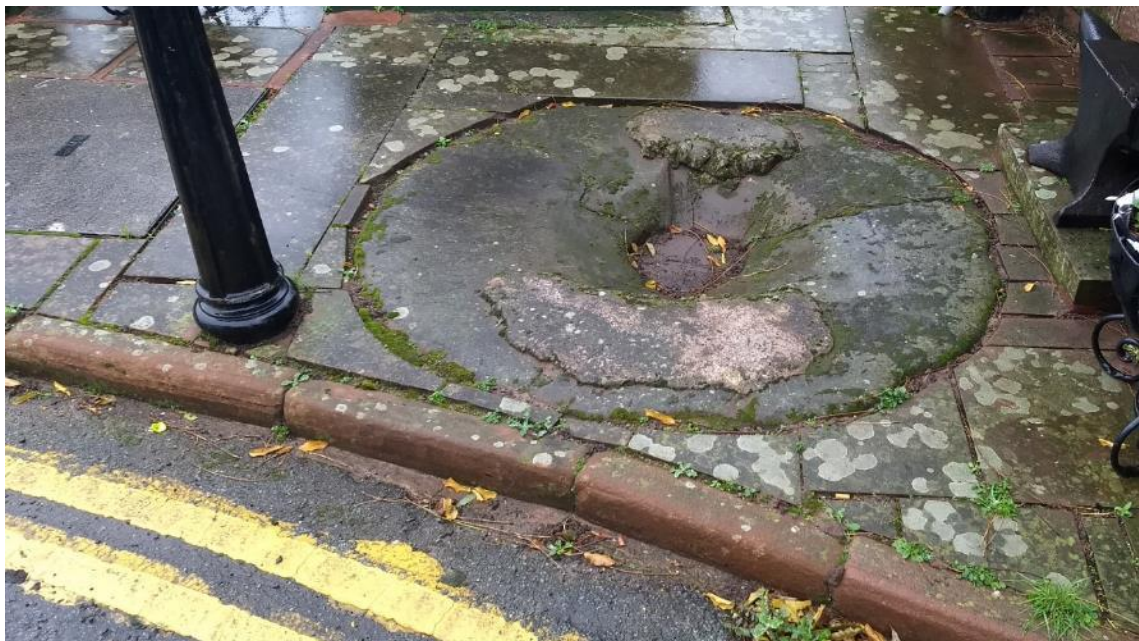
Figure 96 This area of pavement at the end of Cross Hill has an attractive flagged surface and, interestingly, red sandstone curbs that add a strip of colour along the edge. Being quite soft, red sandstone is not commonly seen as a curbing material.
