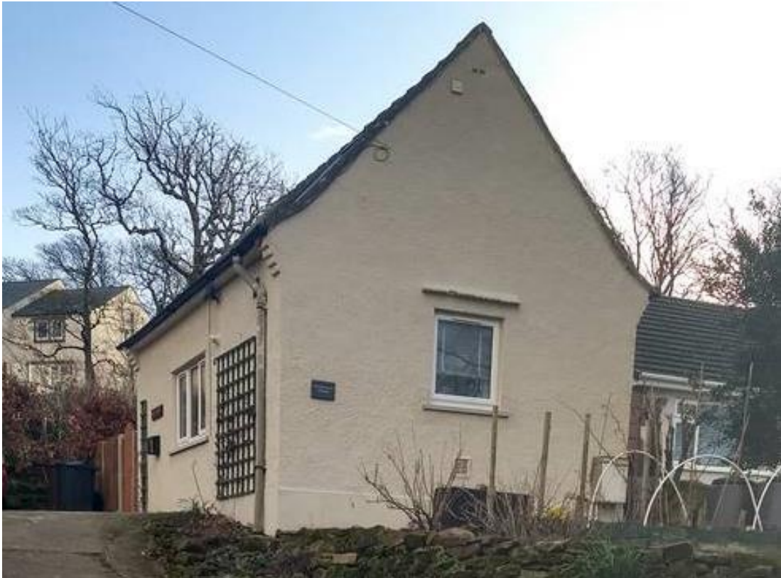
Figure 42 The Old Telephone Exchange
