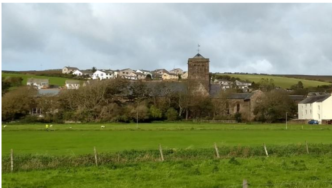
Figure 7 The setting of the priory church has been harmed by post-war housing that not only lacks architectural merit but is positioned on a hill so as to be visible from the entire surrounding area.
