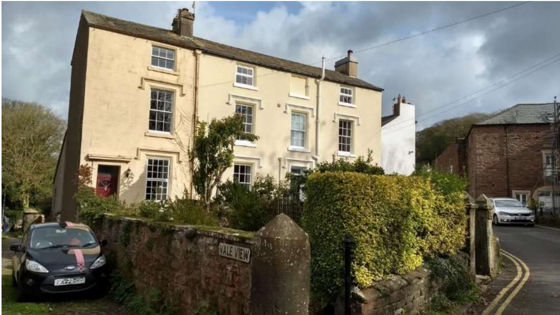
Figure 45 Mayfield, a very elegant grade II listed house dating from the 19th century. The irregular arrangement of plots, interspersed with mature planting and beautiful boundary treatments, are what gives this character area its nature.
