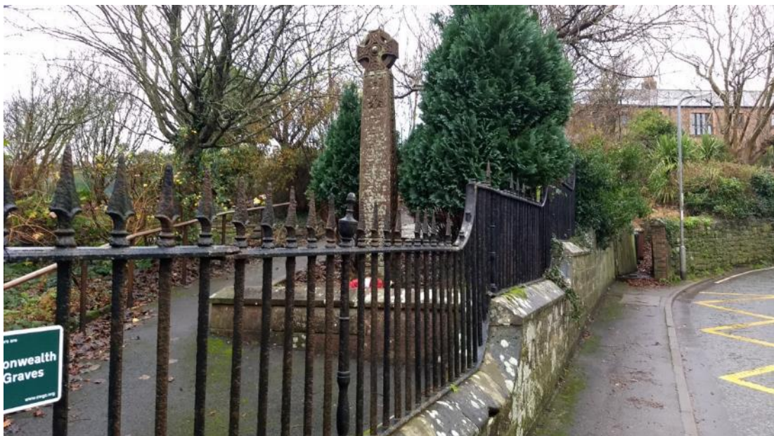
Figure 16 Historic iron railings have survived near the priory lych gate, although one or two finials have been broken off. This photo also shows the earlier of the two WWI memorials. WWII names were added below on an engraved stone.
