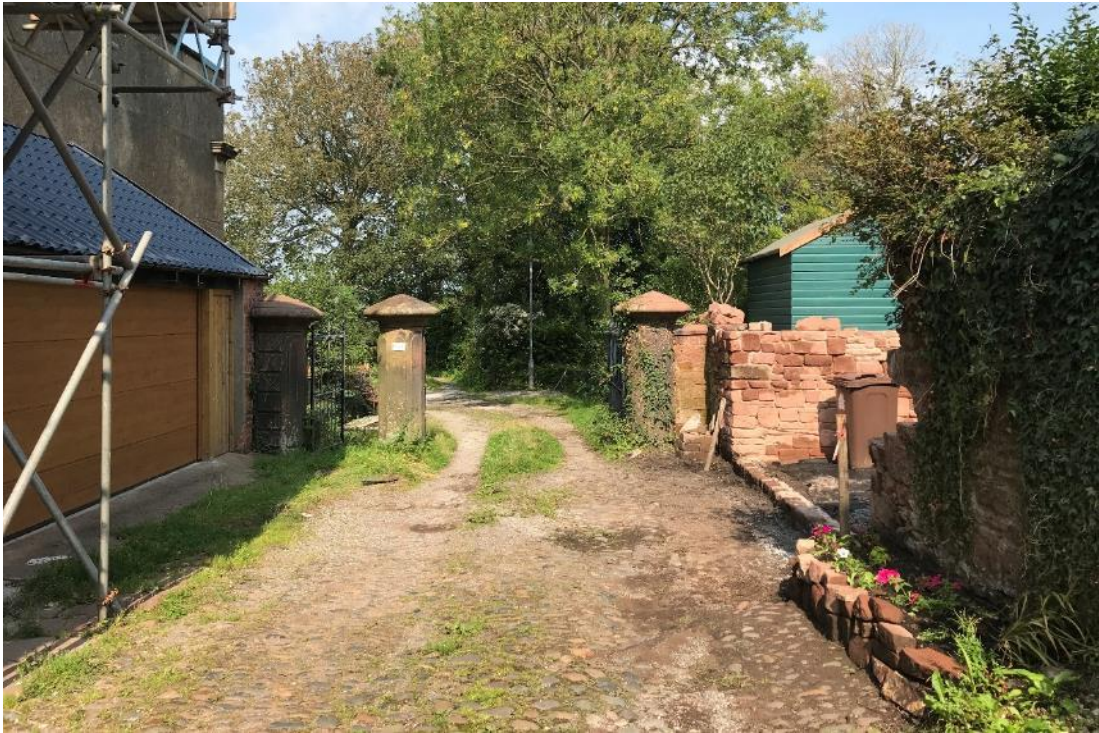
Figure 46 The distinctive piers dividing the two sections of Vale View. Note also the cobbled surface, which appears to have been damaged by the passage of heavy vehicles.
