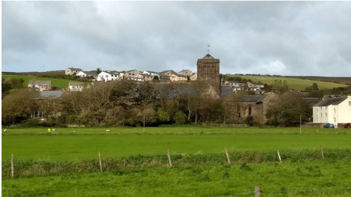
Figure 84 In places, the green surroundings have been lost, though this is fortunately fairly minimal
