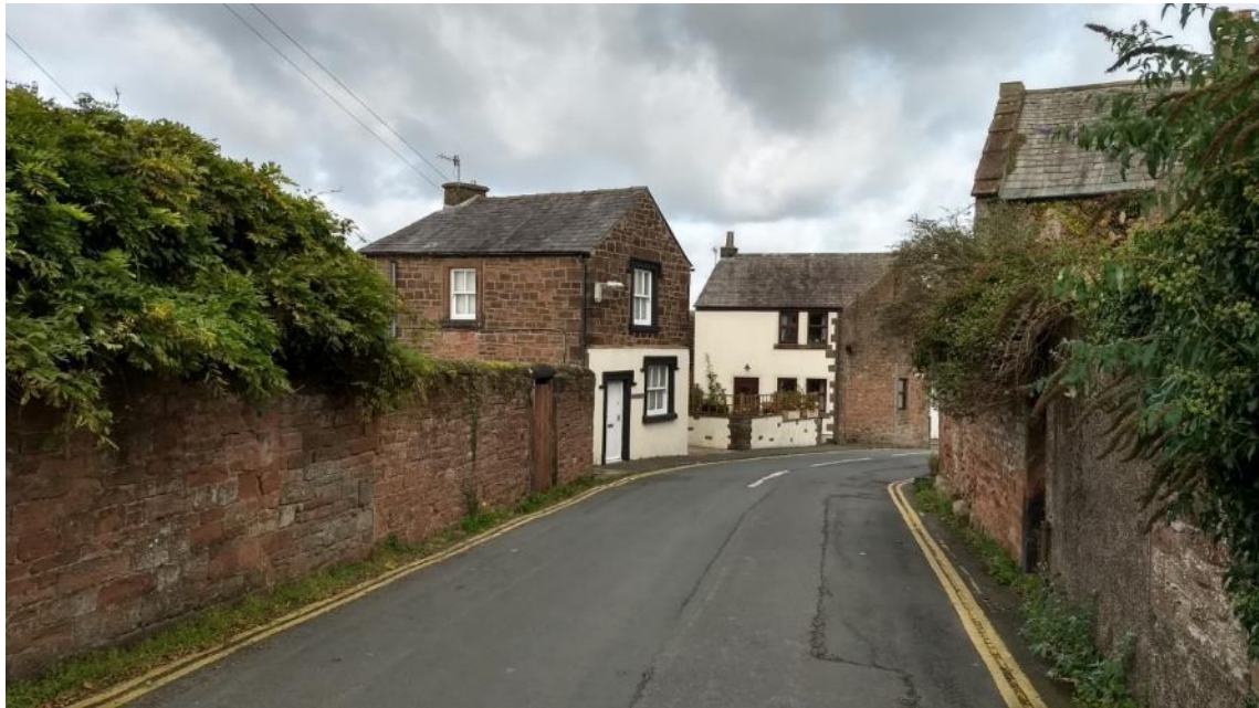
Figure 78 Red sandstone on Cross Street (Thimble Cottage in the centre), creating a wonderful richness and softness in combination with vegetation, slate roofs, and timber windows.
