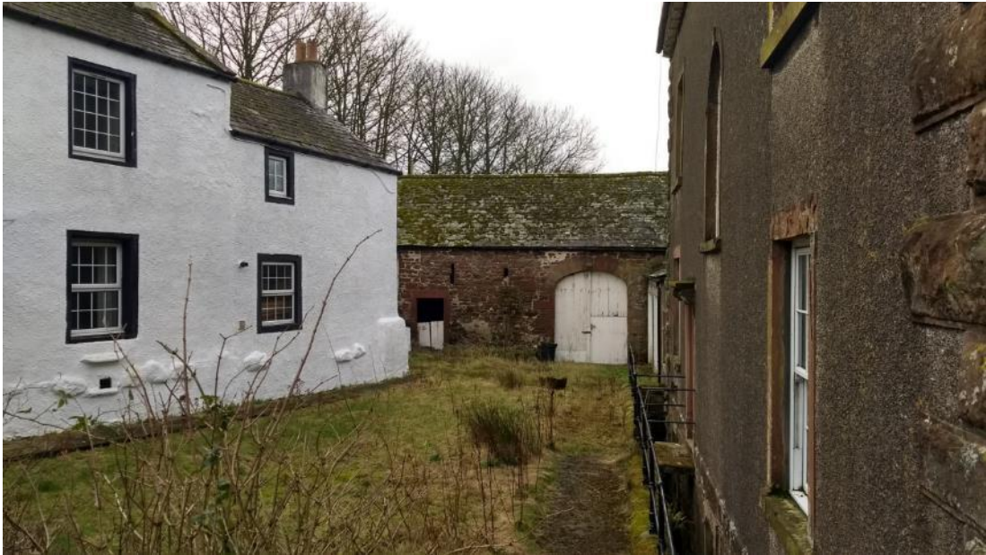
Figure 31 A cluster of historic buildings at the north-eastern corner of the conservation area on High House Road
