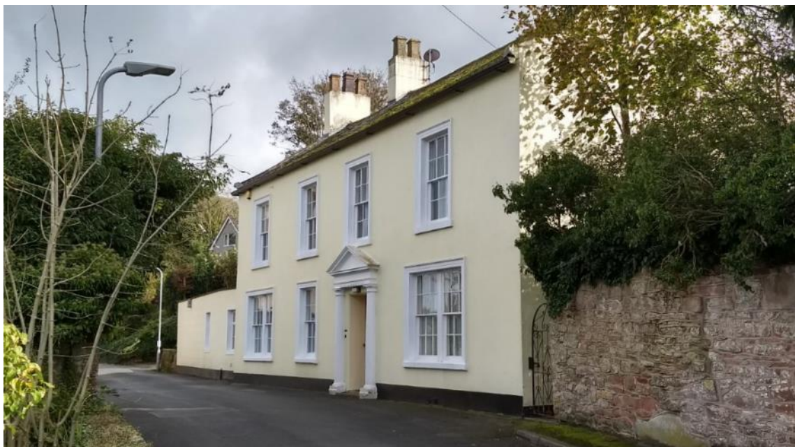
Figure 82 Timber sash windows have generally been one of the heaviest casualties in St Bees, however, where they are retained (even in a somewhat anachronistic brilliant white colour) they complement the area. Much can be done to improve the performance of timber single-glazed windows, and where renewal is necessary a suitably specified double-glazed example is often acceptable, and provides a balance between insulation and appearance.
