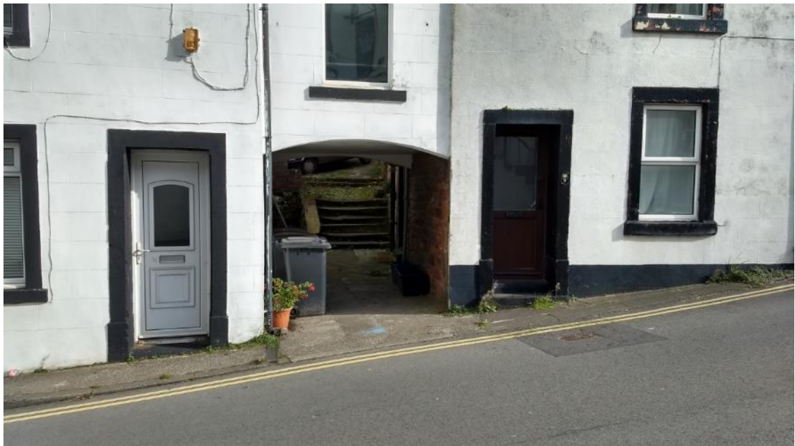
Figure 91 Surviving carriage arches such as this one on Main Street provide a glimpse into the semi-hidden spaces behind.
