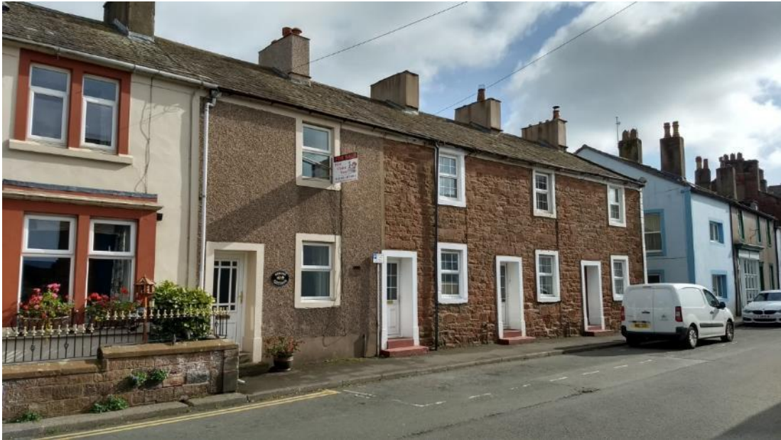
Figure 61 Sandstone cottages typical of Main Street: simple in appearance, two storey, and fronting the pavement. Though there are plenty of cottages like this on Main Street, the area's variation is one of its strengths. Note the completeness of the chimney stacks, an important detail, even if many are missing their pots.
