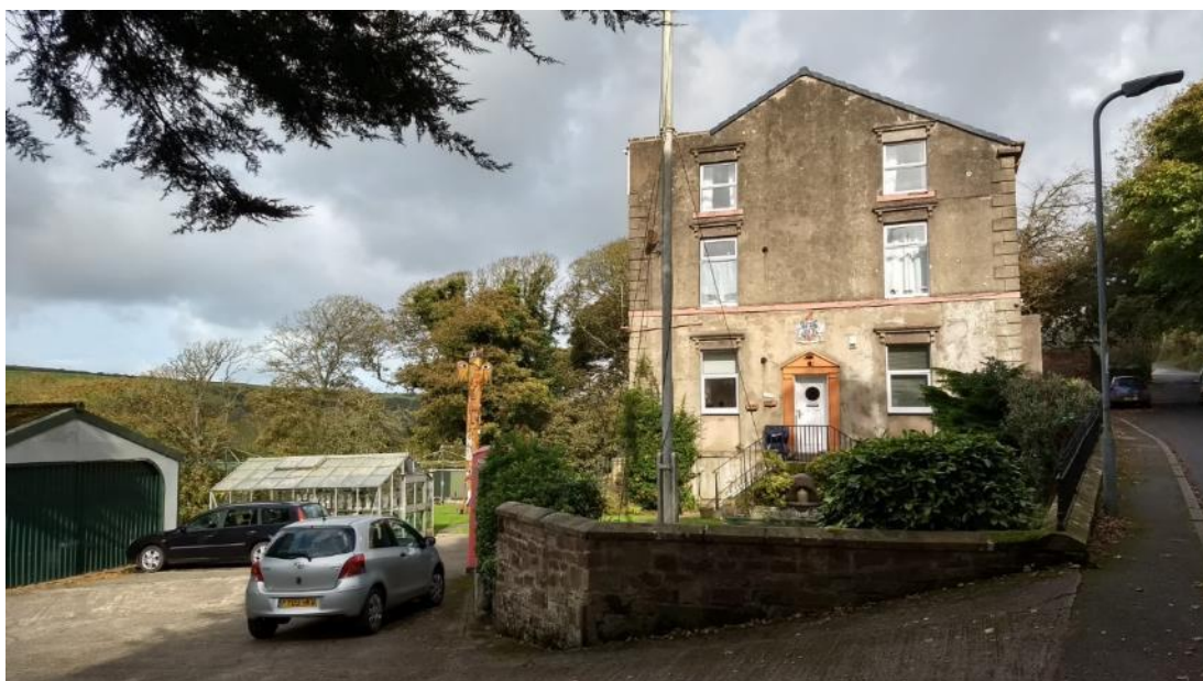
Figure 34 Meadow House, converted to flats, with unsympathetic dormer and plastic windows. There is also a K6 telephone box (one of at least three in St Bees), which appears to have been moved here as an ornament.
