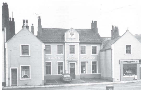
Railings removed and wings increased in height 1950
