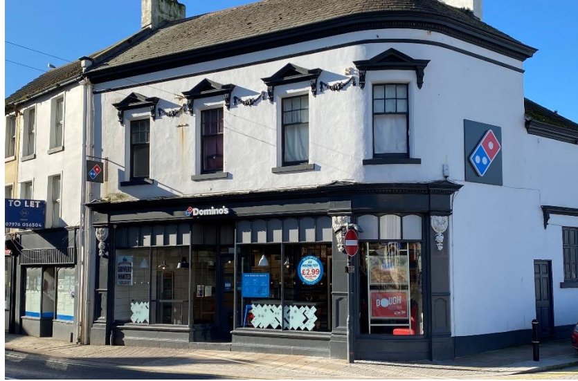
Figure 33 This building on Tangier Street, Whitehaven, dates from the turn of the 19 th /20 th centuries. It retains almost all of its original detailing, including this excellent shop front.
