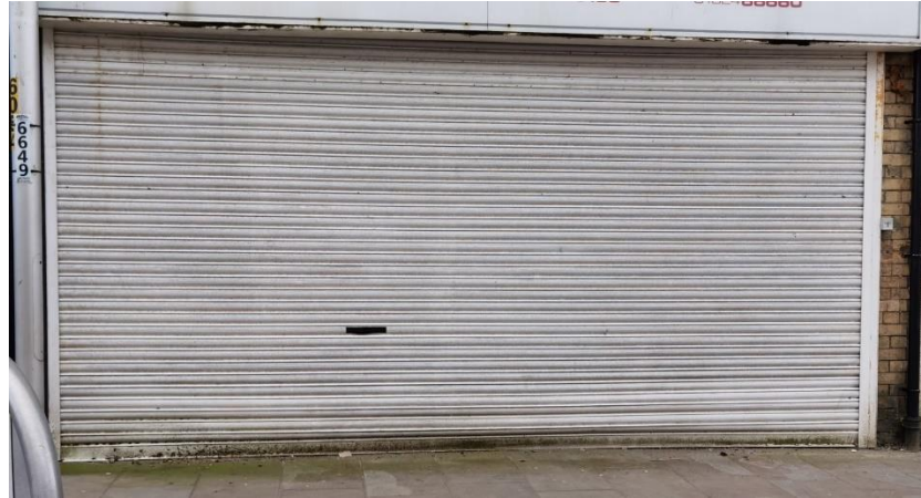
Figure 23 Heavy-handed external shutter. This projects a poor appearance when closed and necessitates the fitment of bulky housings for when it's rolled up.
