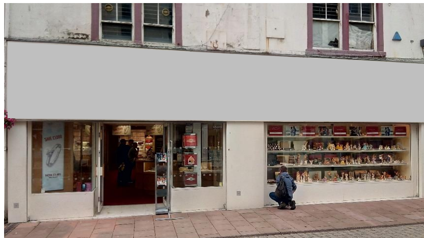
Figure 15 This fascia is oversized. It occupies almost half the vertical height of the shopfront.
