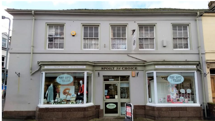
Figure 27 This shop on Lapstone Road in Millom is unusual in being fronted by a pair of canted bay windows.
