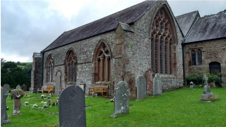
Figure 9 Holy Trinity Church from the south. The graveyard contains stones from a number of centuries, as well as a chest tomb and sundial that are listed in their own right.
