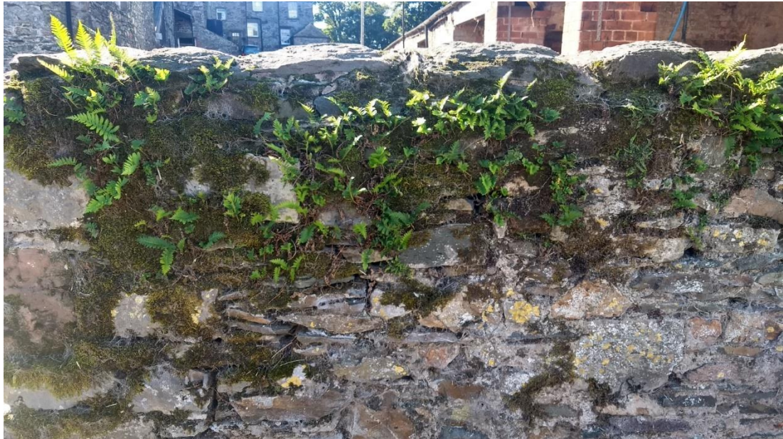
Figure 13 The old rubble wall at the roadside
