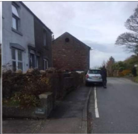
Above - B5344 west of HDH1 site – narrow and sometimes blocked pavement
