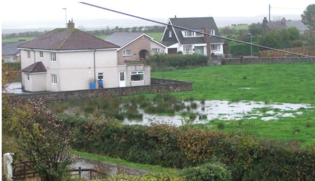
Figure 8 Flooding in land to which the application relates on 14 October 2018 (Date stamped on camera)
