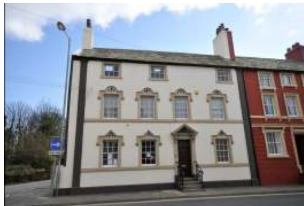
Trinity House, Irish Street – Traditional materials used in the Georgian buildings of the town centre include rendered stone rubble walls, stone door and window surrounds and wooden window frames and doors
