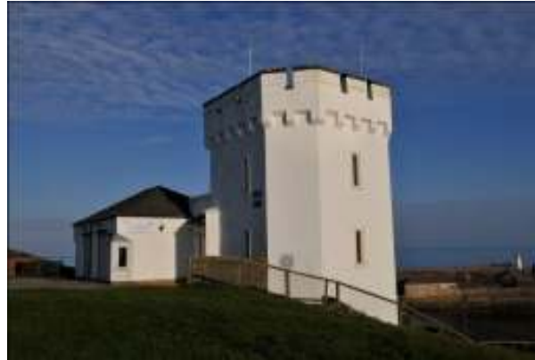
Wellington Lodge – The use of rendering gives added protection to the building in its exposed harbourside location
