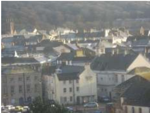
Roofscape looking East across town centre
