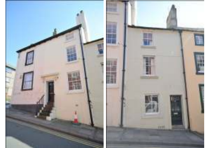
Scotch Street – Buildings "step up" the hill side
