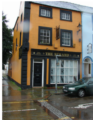
Inappropriate use of colour
