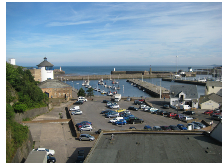
View from the south
