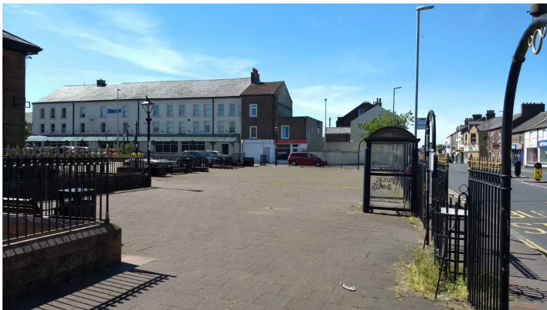
Figure 39 Edges in Market Square are characterised by slightly haphazard and untidy collections of fencing, bollards etc. These are not optimal.
