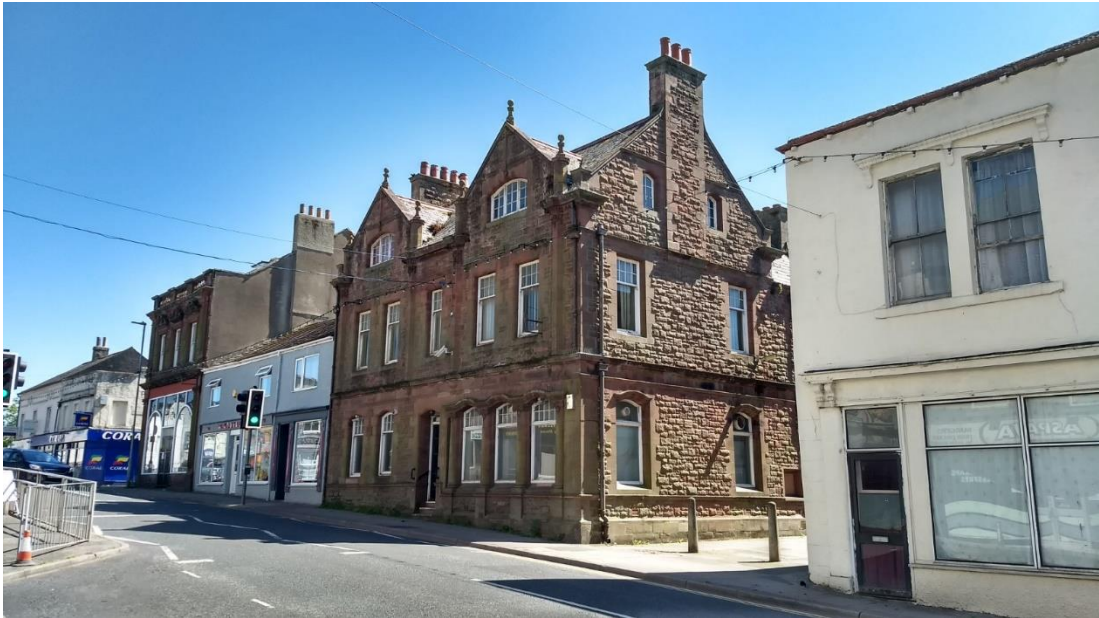
Figure 30 The grade II listed former Natwest at 58 High Street
