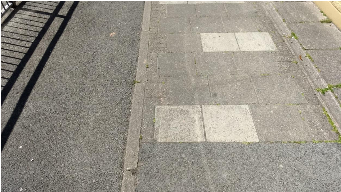
Figure 37 Concrete and tarmac surfaces abound
