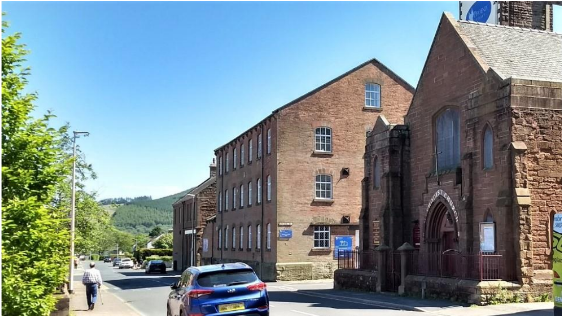
Figure 17 Methodist church and Phoenix Court
