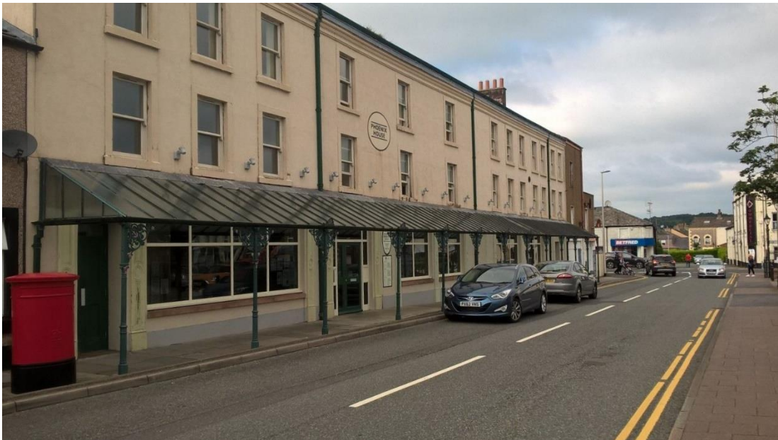
Figure 14 5 Jacktrees Road and its veranda, listed Grade II
