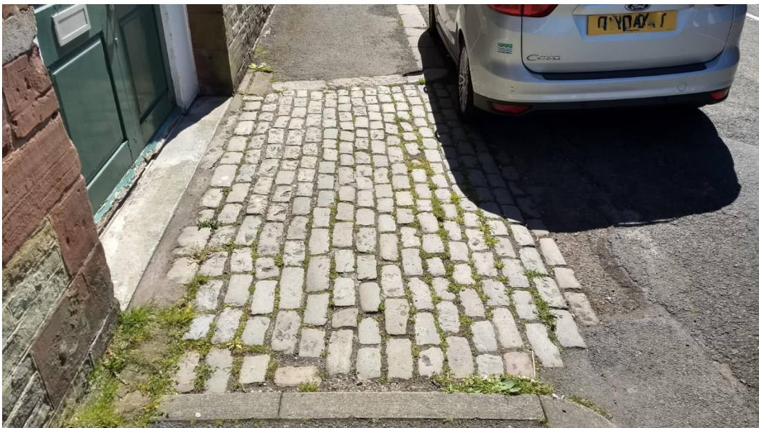
Figure 38 An area of original stone setts outside a door at Phoenix Mill on Ehen Road. This is one of very few original areas of surfacing left
