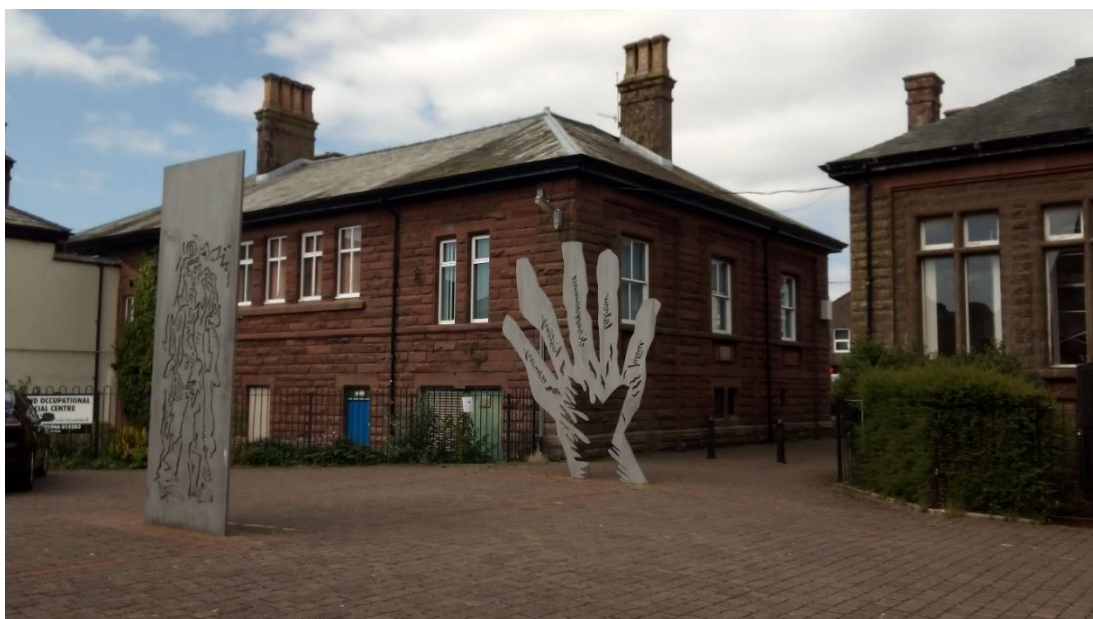
Figure 8 Local Government Offices, listed grade II, along with two of the Square's three sculptures by local artist Conrad Atkinson (1988).
