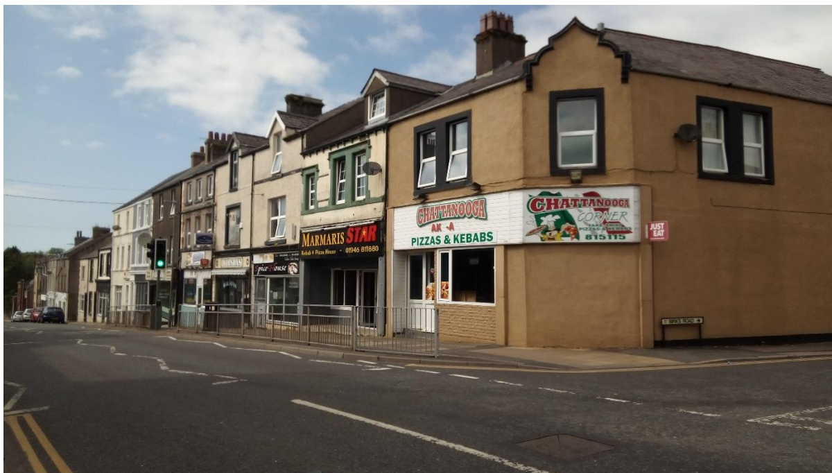
Figure 42 High Street looking to the west, showing unsympathetic fenestration, loss of shop fronts and unattractive signs. Note also the nearest building, which has lost its corner doorway at some point, upsetting the emphasis of its façade. The streetscape is particularly uninspiring, comprising tarmac, concrete and steel, none of it deployed with any thought for attractiveness.
