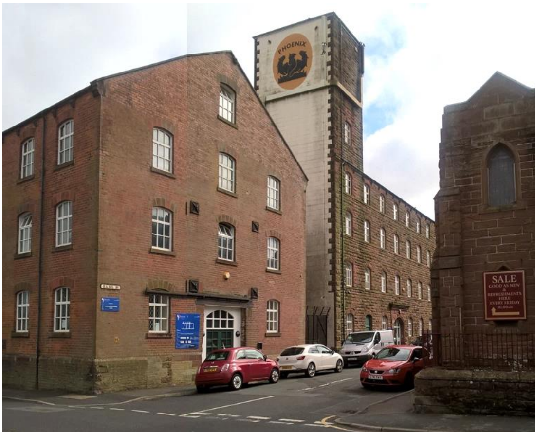
Figure 19 The former flour mill on Earl Street
