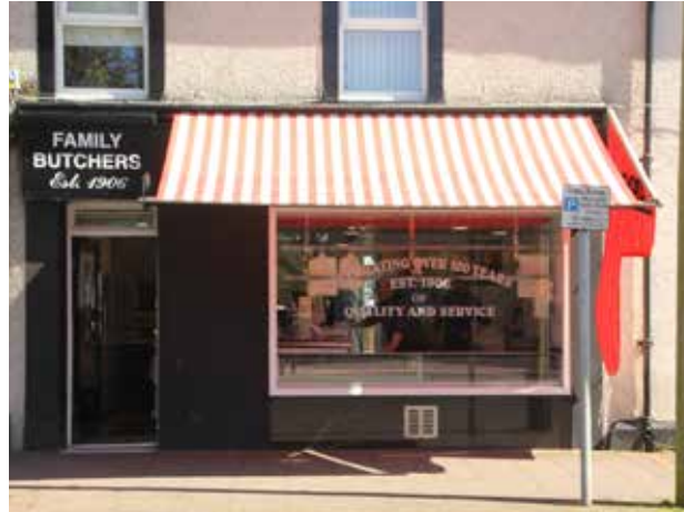
A straight, canvas awning with lattice strut mechanism is a traditional feature in a conservation area.
