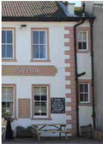
Discreetly sited retrofit soil vent pipe, with decorative terminal.
