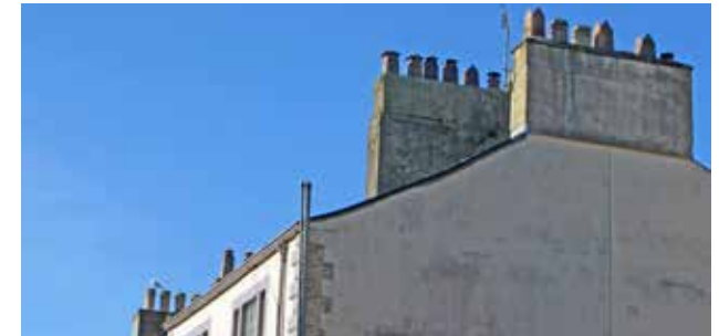
Chimneys stacks on terraces often serve the fireplaces in two houses, so are quite substantial with a large number of pots.
