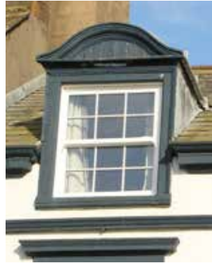
Traditional Victorian dormer with lead clad cheeks.
