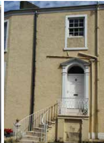
This retrofit foul drainage installation pays no regard to the proportions of this period elevation.
