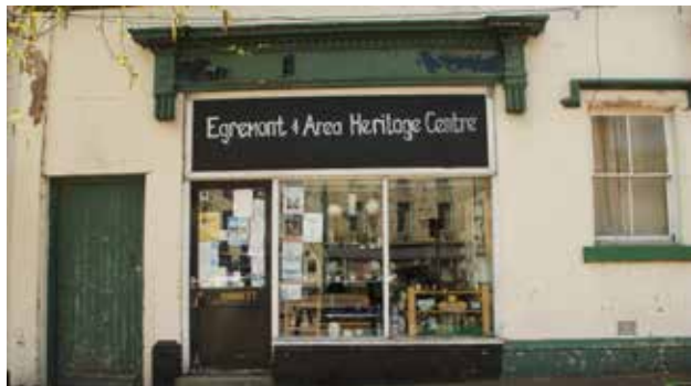
Loss of historic features: pilasters each side of shopfront have been removed and the sign spoils the proportions of the shop window instead of occupying the traditional fascia above.
