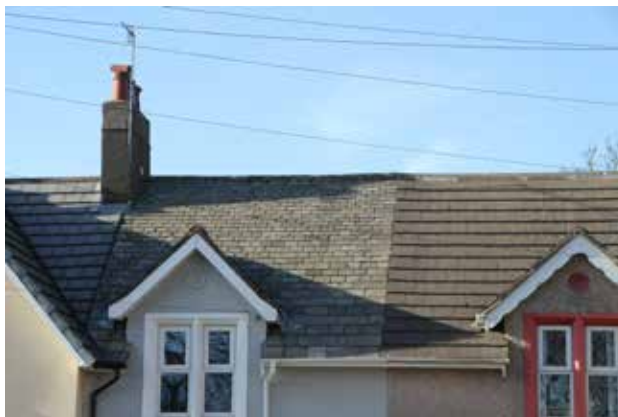
Westmorland slate roof, with roofs on either side replaced in tiles.
