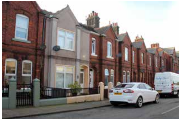
This terrace of houses in Millom is decorated with brick detailing. The second house from the left has been rendered in an inappropriate dash finish burying the brick detailing.
