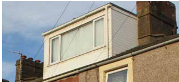
A flat roofed dormer with horizontal timber cladding 'perched' upon a traditional roof pitch.
