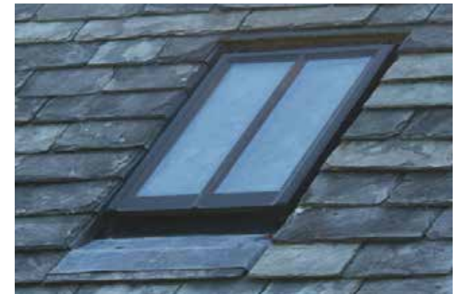
Conservation rooflight - small unit with vertical emphasis and low profile flashing kit, sits flush in the roof plane.
