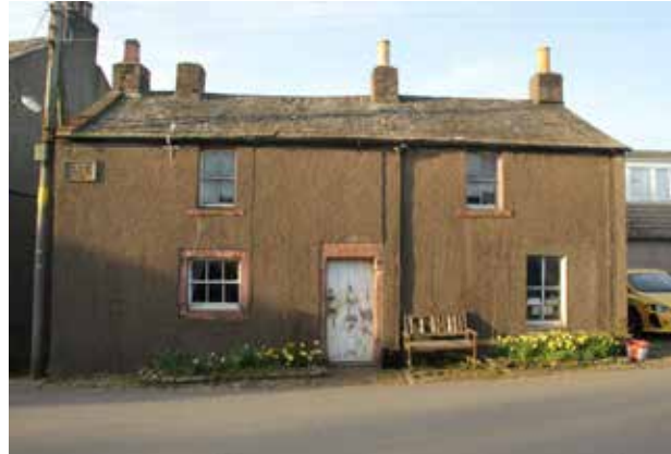
The appearance of this traditional building has been spoiled by the retrospective application of roughcast render, which protrudes beyond the sandstone dressings.
