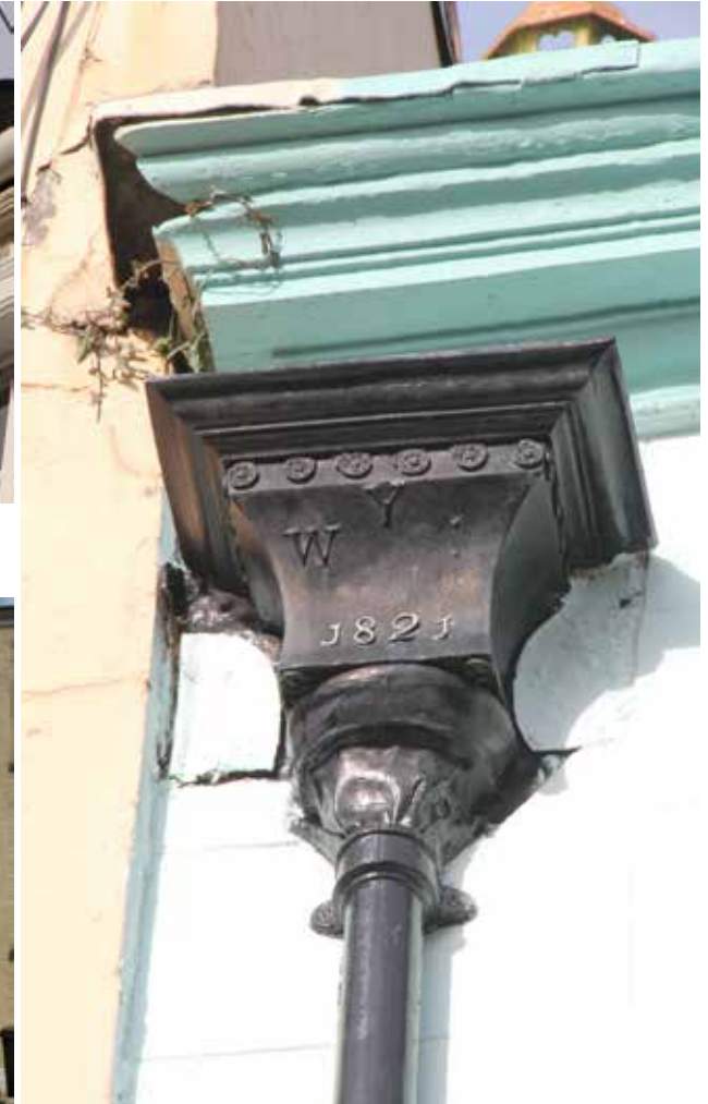
Ornamental copper rainwater hopper, discharging into a cast iron rainwater pipe.
