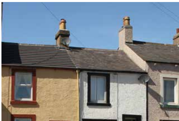
Welsh slate roofs with roof on left replaced in tiles.
