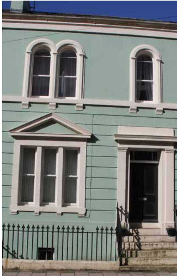
Rusticated finish to ground floor masonry, with deeply incised horizontal lines.
