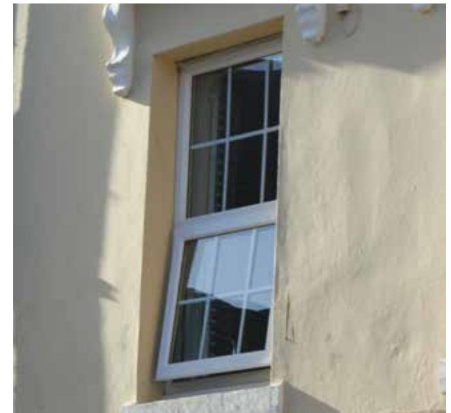
A uPVC replacement window with broad flat frames and an alien opening light arrangement.
