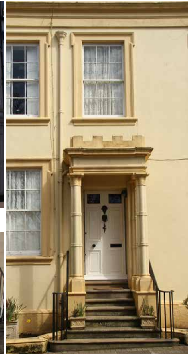
When rainwater pipes are painted the same colour as the wall upon which they are fixed, it reduces their impact.
