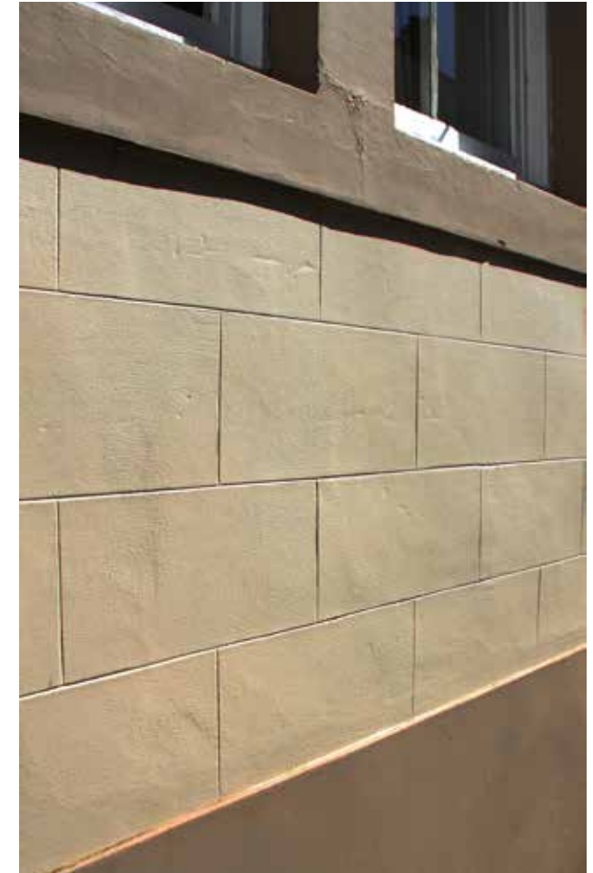
Incised lining on stucco to appear to be ashlar masonry.
