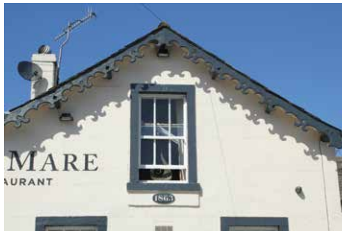
Floodlighting tucked under bargeboards achieves the objective of lighting the elevation, without the light fittings themselves being conspicuous.
