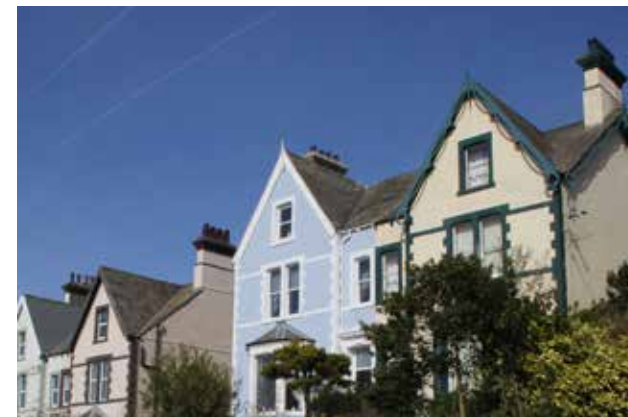
Original decorative bargeboards on right hand gable. Bargeboards to left are simple 'plank' replacements.
