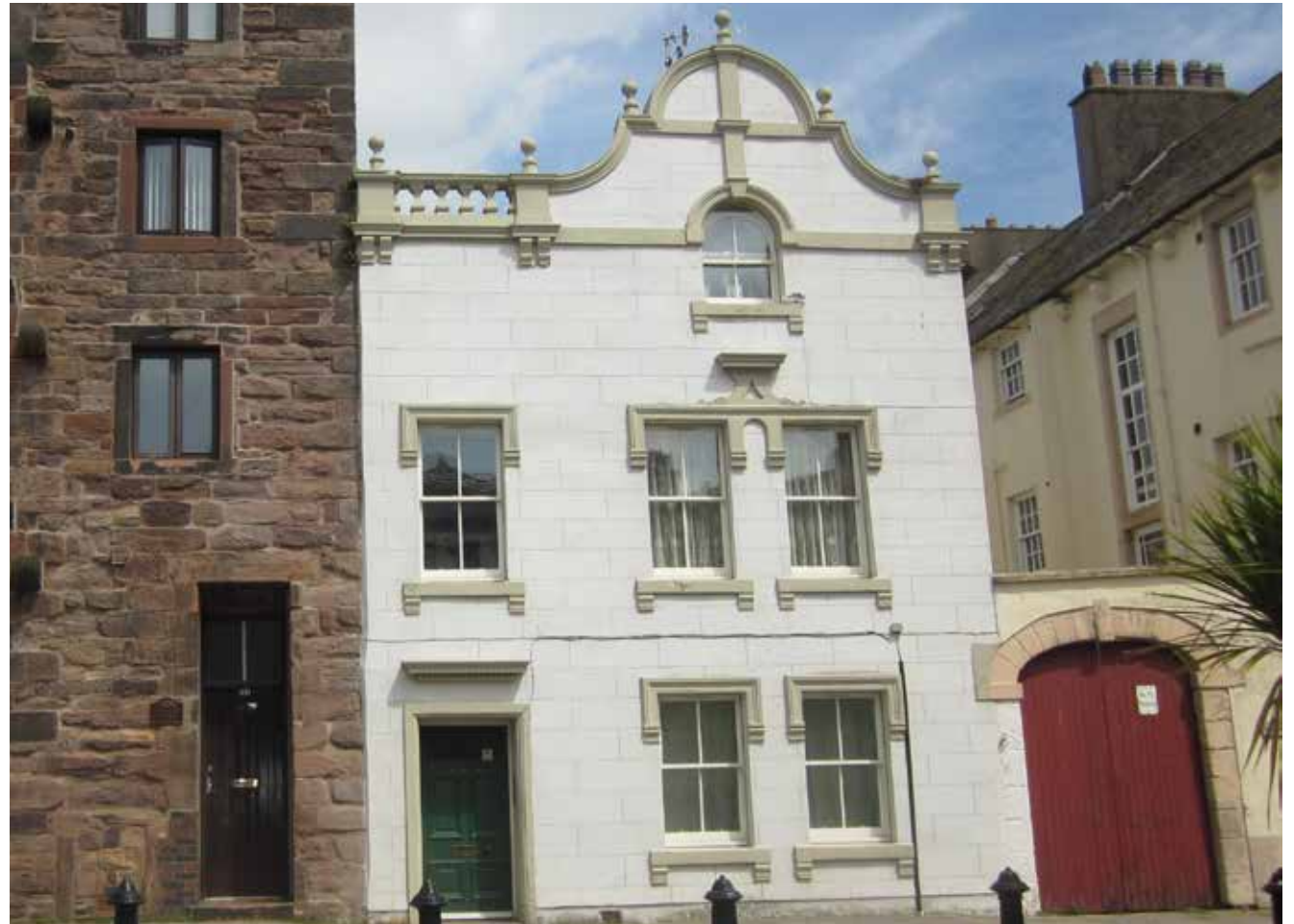
Restored Dutch gabled listed building in Roper Street, Whitehaven, with new windows, external render & refurbished front door.
