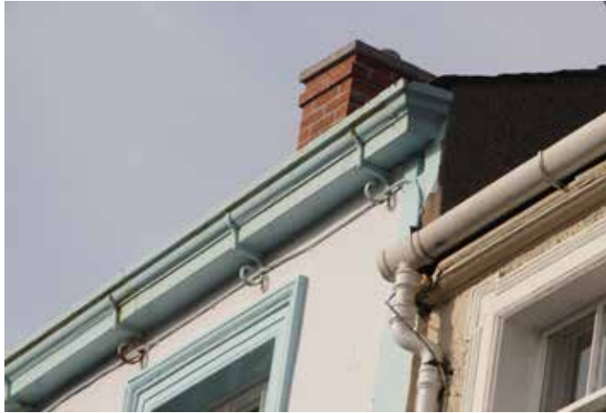
Traditional ogee profile cast iron gutter, supported on decorative cast iron gutter brackets.
