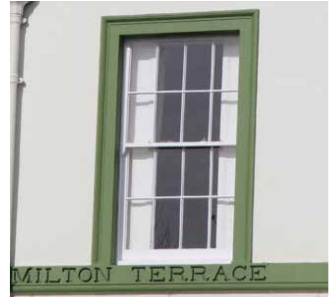
An example of a late Georgian double hung sash window.
