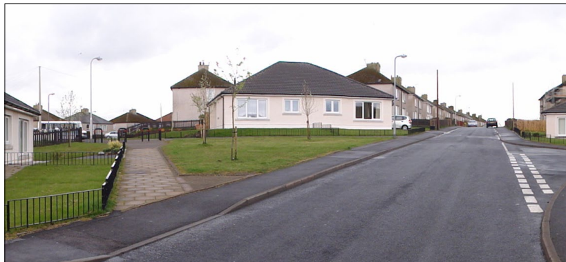
Some improvements to properties, boundaries and front garden areas have already been undertaken by Home
