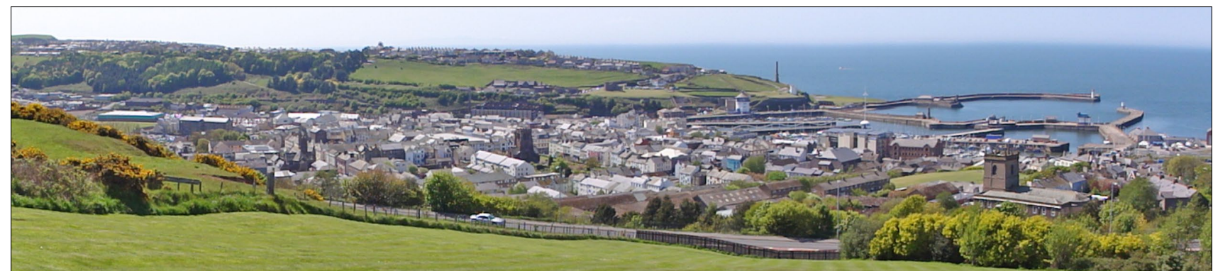
Panoramic view over Whitehaven from 'Highlands'. A predominantly render town in terms of materiality and form. Woodhouse and Kells sit on top of the far left ridge line accessed via the distinct Ginns to Kells Road
