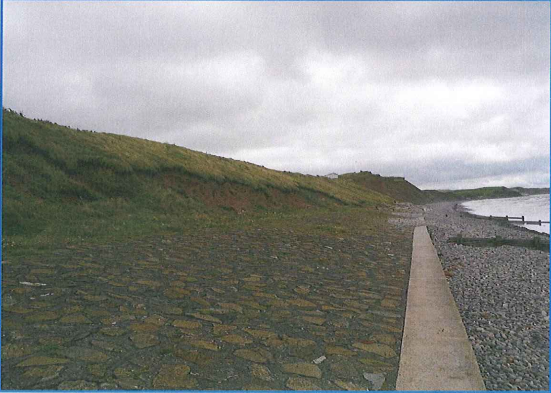
St Bees foreshore looking south
