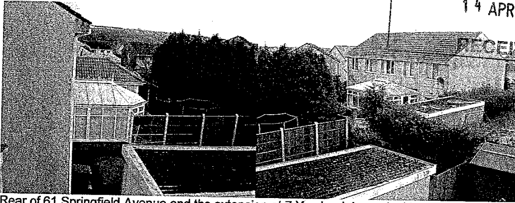
Rear of 61 Springfield Avenue and the extension at 7 Yewbank Lane, looking north-west from 65 Springfield Avenue
