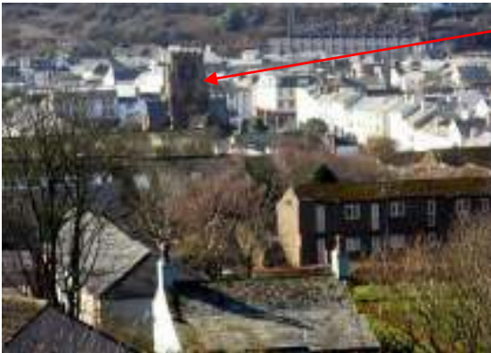
St. Nicholas' Church Tower
