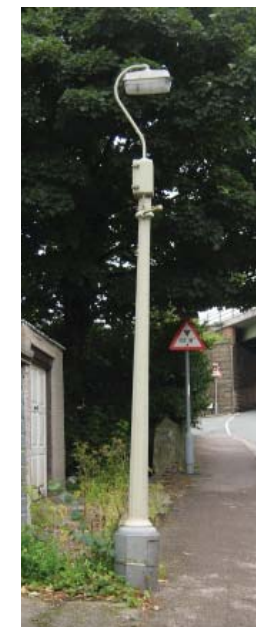
Street lighting column
