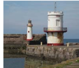
North Pier Lighthouse
