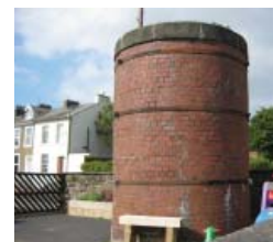
Red brick air shaft cap
