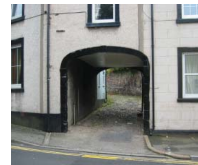
Smoothed stone setts in rear courtyard
