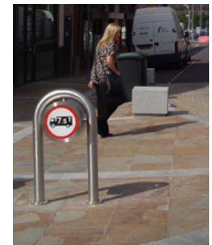
Discreet traffic signage with dual function as bollard
