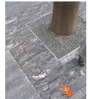
Change of texture around hazards : More London Place, London
