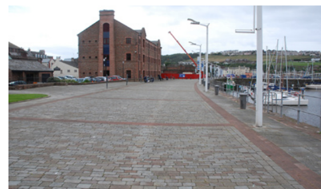
Stone setts to harbour quayside
