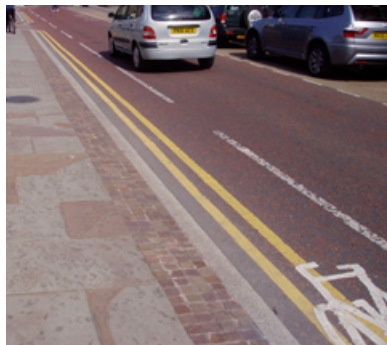
Large, textured random sandstone paving, smaller units to edge and no colouration to cycle way : King Street, Blackburn
