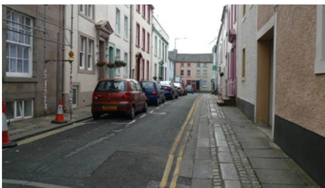
Footway, kerb and channel with high quality sandstone
