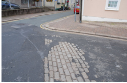
Above: In some areas stone setts still remain under the tarmac.
