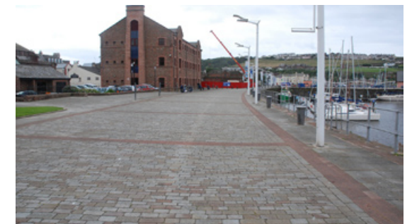
Type 1: Good quality sandstone surfacing to Millennium Promenade
