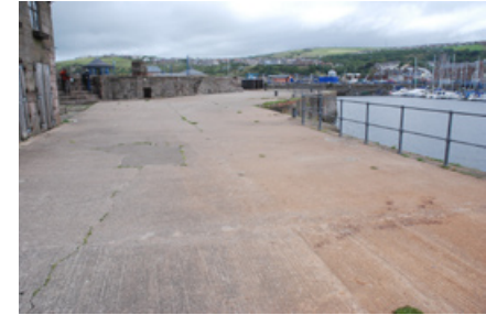
Below: In situ concrete to rest of Northern Pier, (type 12).
