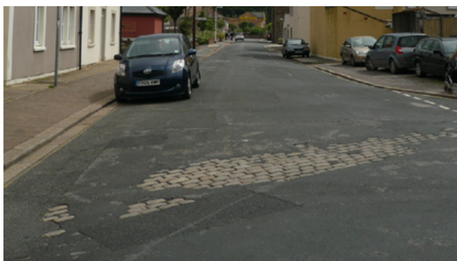
Fragments of traditional materials remaining under tarmac. Large random sized, textured sandstone on footway and sandstone kerb.
