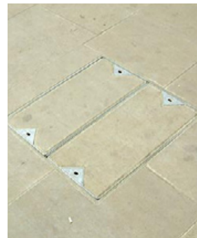
Recessed utilities covers : Kensington High Street, London
