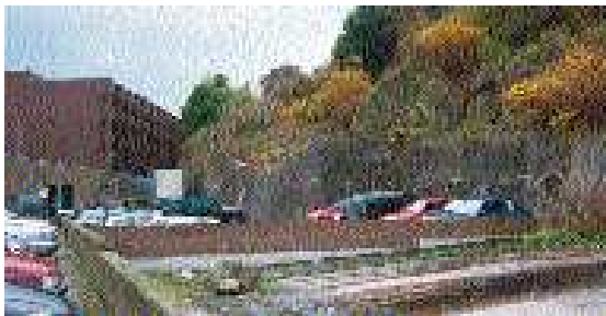
(6) Mountpleasant: remains of old buildings at base
