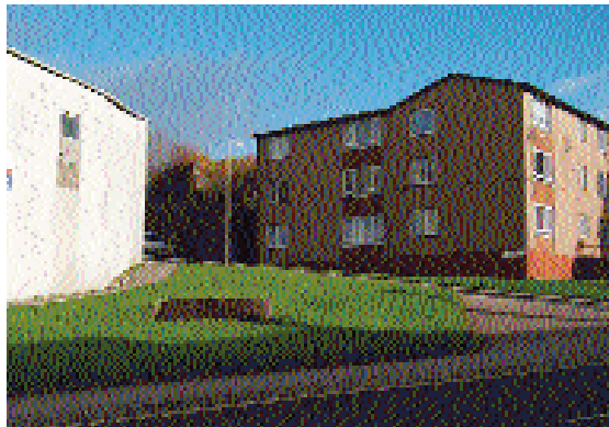
(13) High Street: Wellington Row junction
