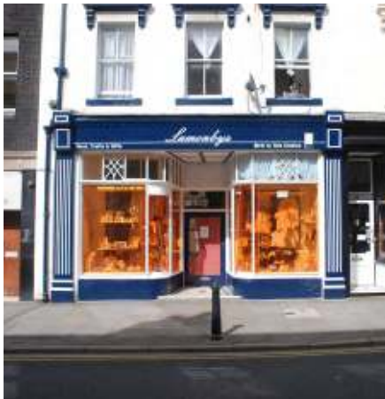
Successful shopfront - retention of traditional frontage, Duke Street
