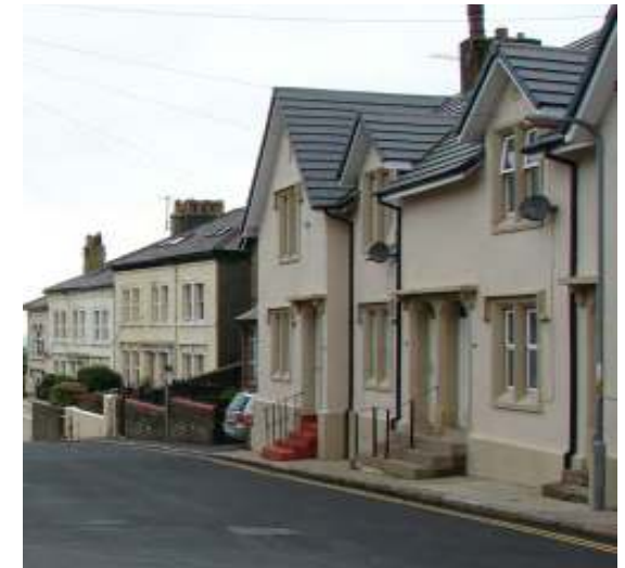
Inappropriate roof repairs, Wellington Row
