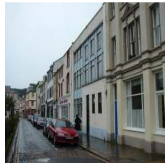
Unsympathetic window alterations using curtain walling, Church Street.
