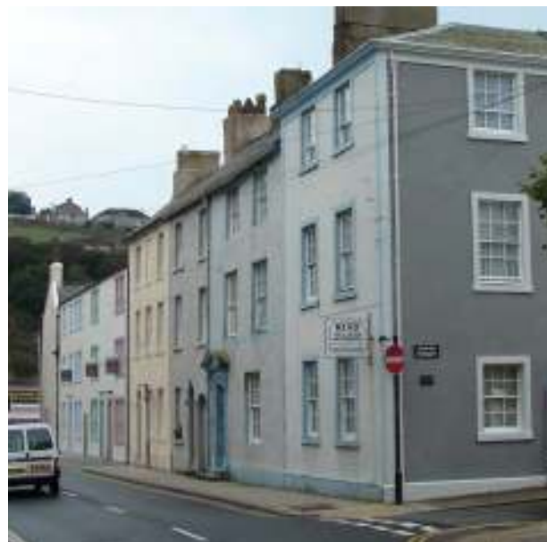
Undulating eaves line to Irish Street
