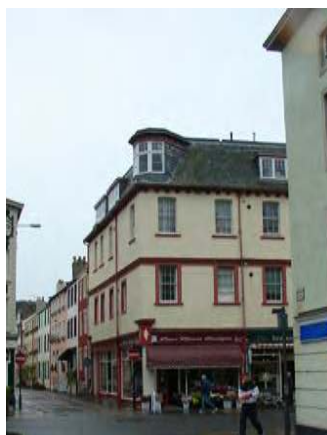
Dormer; Lowther Street
