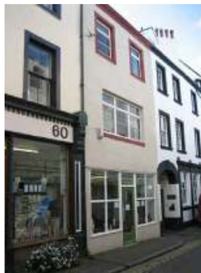
Unsympathetic window alterations to ground and first floors, Roper Street.
