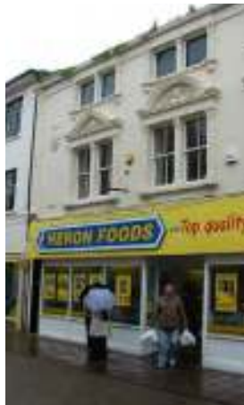
King Street Unsympathetic shopfronts
