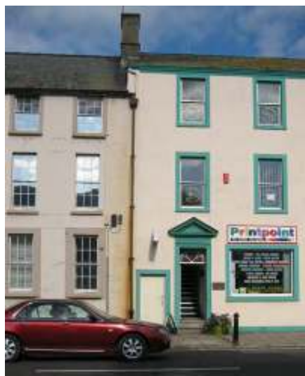
Loss of Georgian astrigals from building on right, Duke Street.
