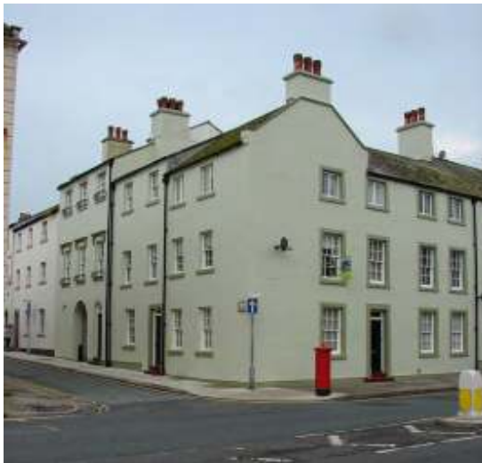
Simple gutter and verge details, Cross Street
