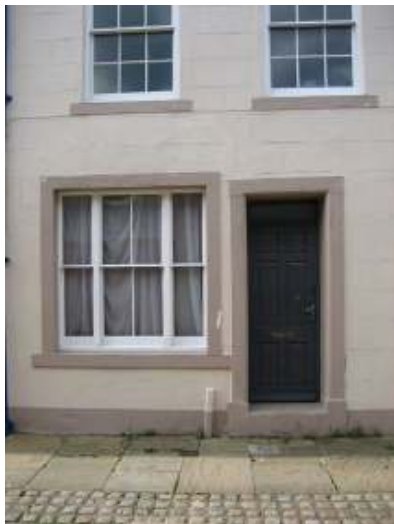
Simple entrance with stone surround, New Lowther street
