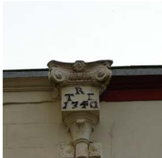
Rainwater hopper, Roper Street
