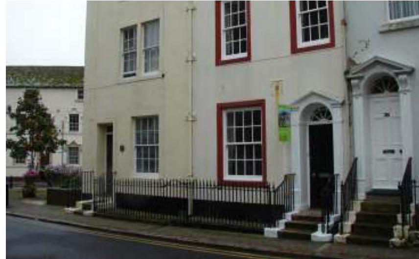
Preserved railings, Roper Street
