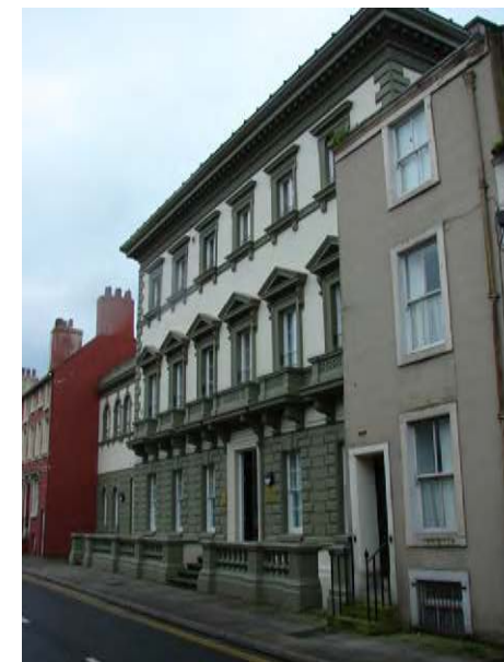
Parapet eaves, Irish Street
