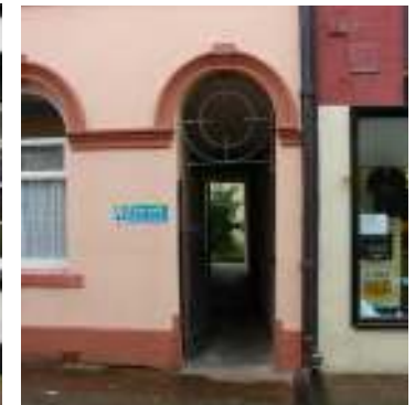
Pedestrian entrance to courtyard, Roper Street
