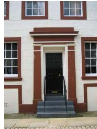
Raised entrance with classical treatment, Church Street
