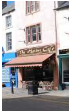
Successful shopfront - use of traditional awning, Duke Street
