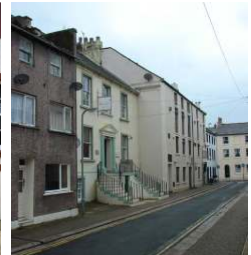
Elaborate stepped entrance
