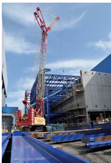
Completing key constructions to cost, time and quality depends on robust project management.
