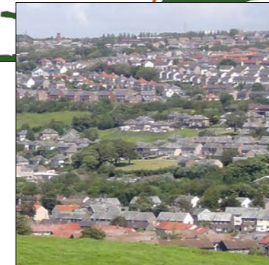
Landscape and roofscape - the 'tiering' effect of much development in and around Whitehaven
